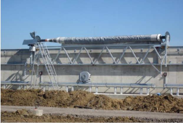
Figure 5. Membrane winding machine, composting plant Hunedoara/Romania
