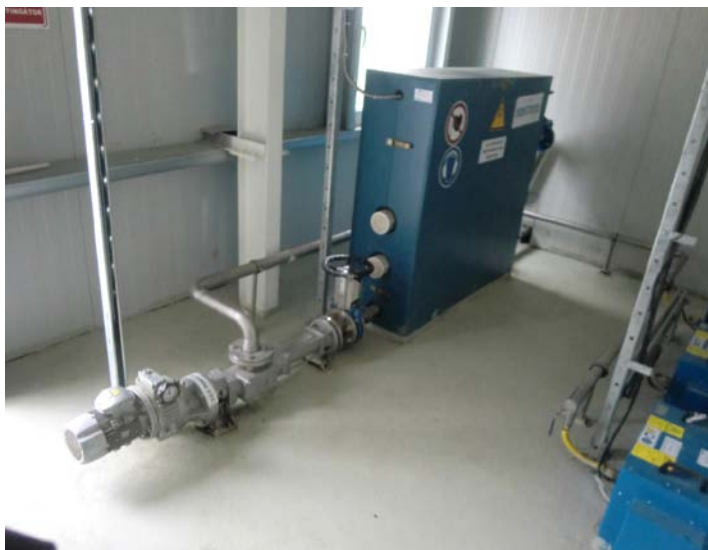
Figure 4. Ultrasonic disintegration installation at Targu Secuiesc WWTP
