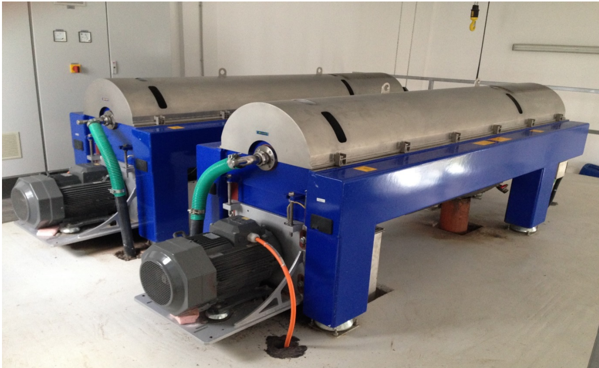
Figure 1. Dehydration unit with gravity discharge of supernatant and sludge
