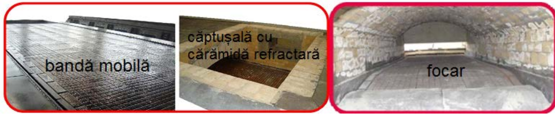
Figure 13. Inside heating plant
