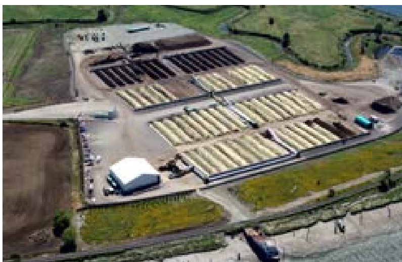
Figure 5. Platforms for sludge composting using semi-permeable membranes
