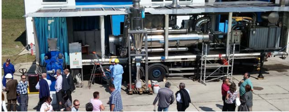
Figure 27. Pilot plant for sludge drying→pelletizing
