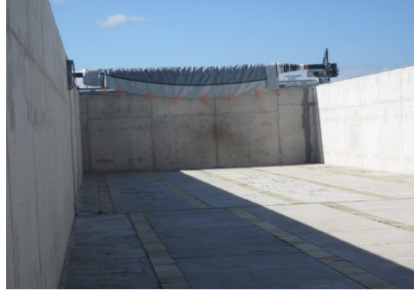
Figure 6. Maximum sized composting box for membrane composting, Hunedoara/Romania
