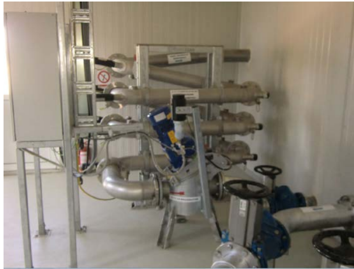
Figure 3. WWTP Targu Secuiesc mechanical and electrokinetic disintegration installation
