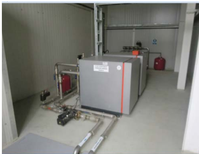
Figure 6. Targu Secuiesc WWTP heat - pump
