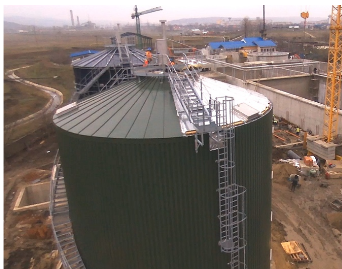
Figure 6b. Anaerobic Sludge Digestion Tank - Vaslui, Barlad
