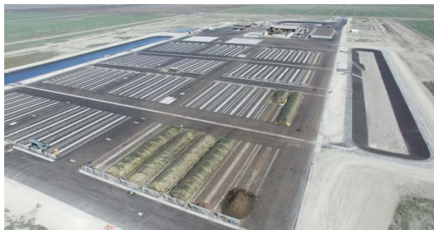
Figure 13. First windrows going into operation for LACSD (total of 72, first stage)
