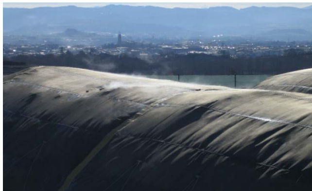
Figure 10. Fervosa plant, distance to next town
