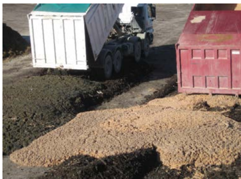
Figure 9. Sludge delivery Fervosa before mixing with structure
