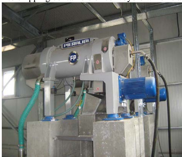
Figure 5a. Dehydration Installation- photo
