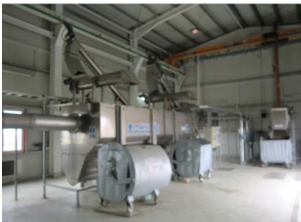
Figure 2. Targu Secuiesc WWTP - Advanced Mechanical Step
