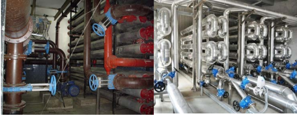
Figure 5. Heat exchangers before and after rehabilitation
