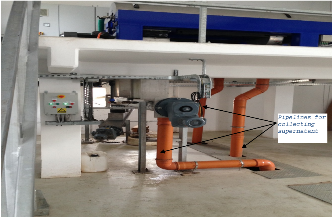
Figure 2. Supernatant collection system, by gravity towards the external supernatant station
