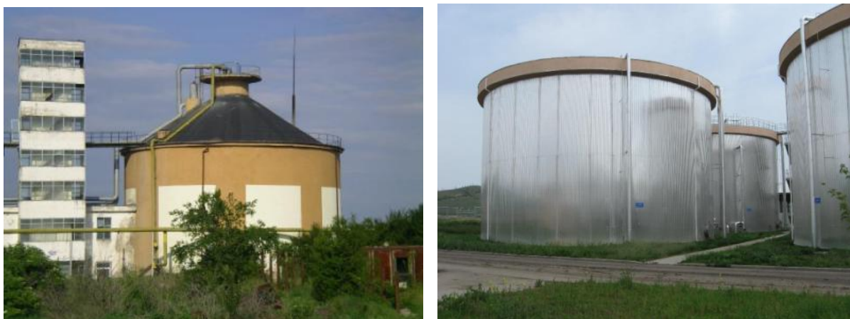
Figure 4. Sludge digesters before and after rehabilitation
