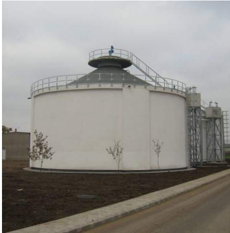
Figure 3a. Rehabilitation Anaerobic Sludge Digestion Tank- foto
