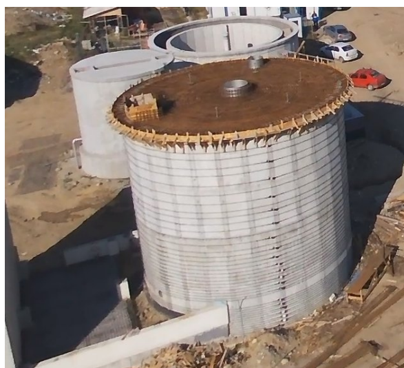
Figure 6a. Anaerobic Sludge Digestion Tank - Odobesti
