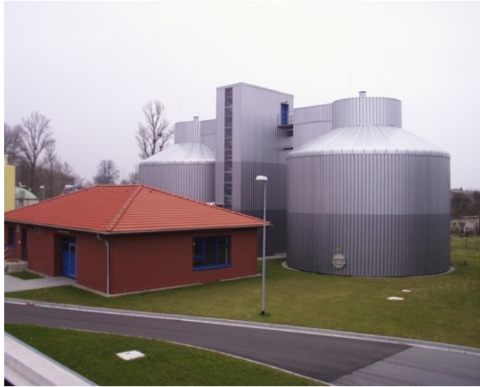
Figure 3. WWTP Stavenhagen/Germany, digesters
