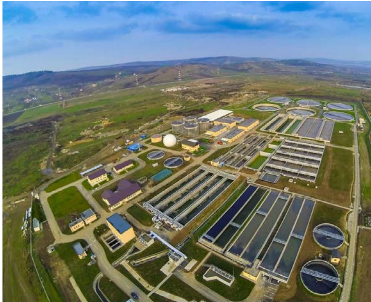
Figure 1. Overview of the Waste Water Treatment Plant
