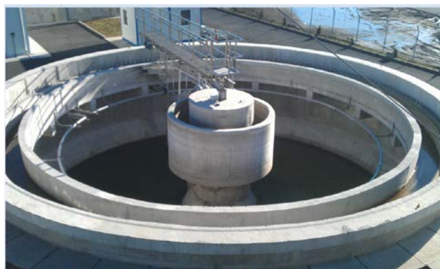
Figure 5. Targu Secuiesc WWTP -Treated water heat recovery installation
