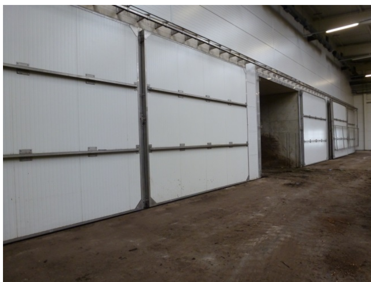
Figure 4. Compost tunnels with gates, view from filling hall, Mondercange/Lux
