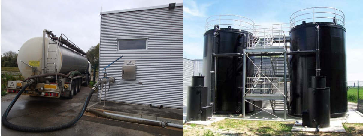
Figure 1. Left: delivery of food waste, station for 24/7 Delivery Right: Tanks for intermediate storage of these wastes
