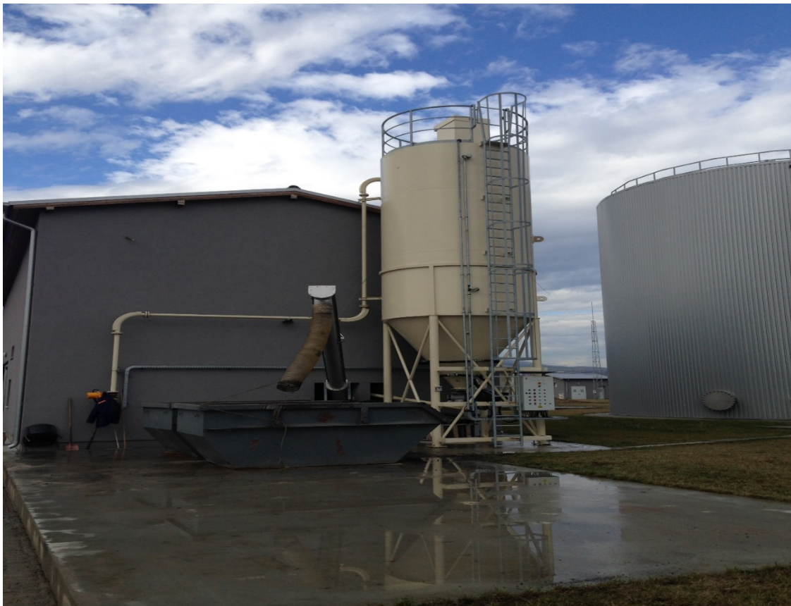
Figure 5. Lime dosing installation
