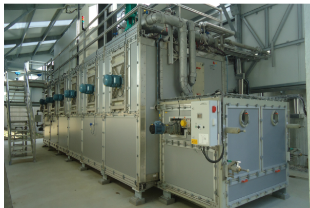
Figure 5. – Photo of installation
