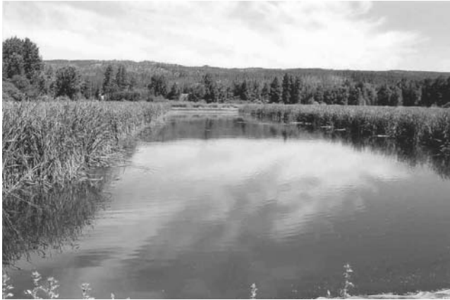
FIGURE 6.4 Free water surface (FWS) wetland at Cle Elum showing bulrush and open water.
