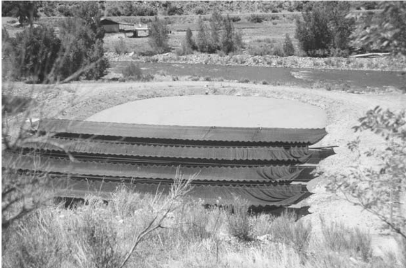
FIGURE 5.8 Photograph of shading for algae control at Naturita, Colorado. (R.H. Bowman, West Slope Unit Leader, Water Quality Division, Colorado Department of Public Health and Environment, personal communication, 2000.)
