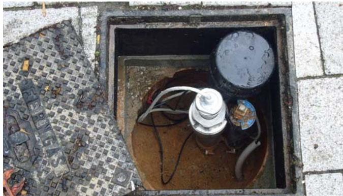
Figure 2: Built-in sluice gate
