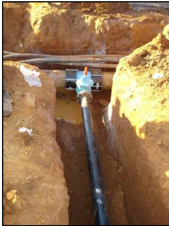
Figure 5: Installation of missing "T-Piece "in Sebokeng
