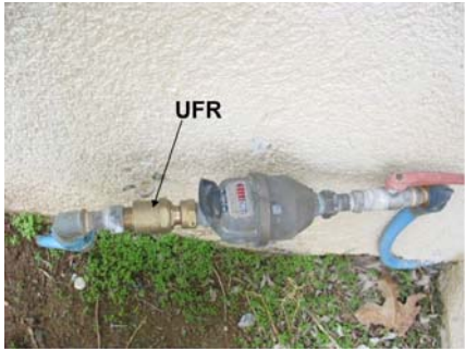
Figure 10. UFR installation
