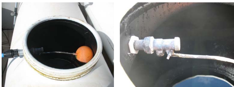
Figure 4. Polypropylene Roof Tank
