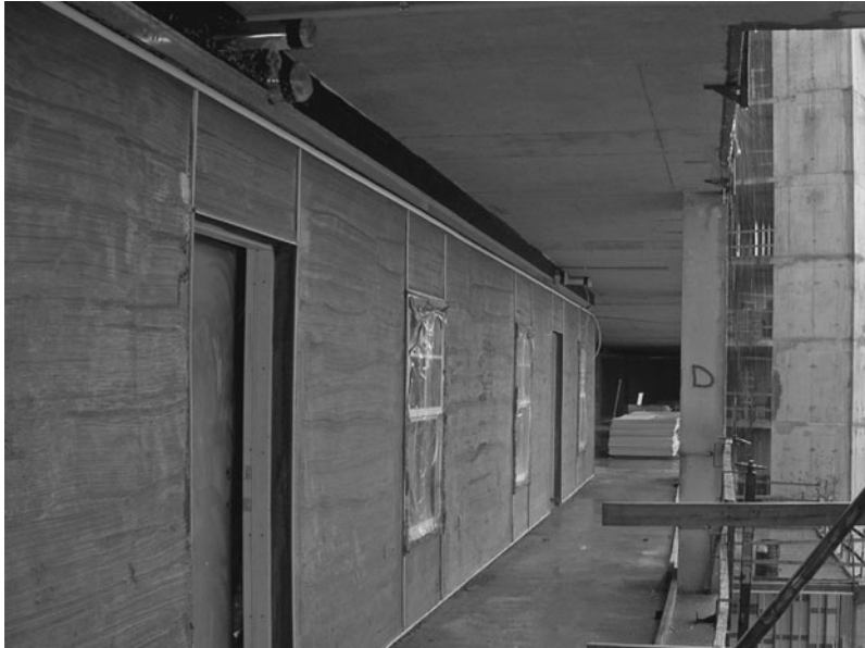
Figure 4-60 Scratch coat.
