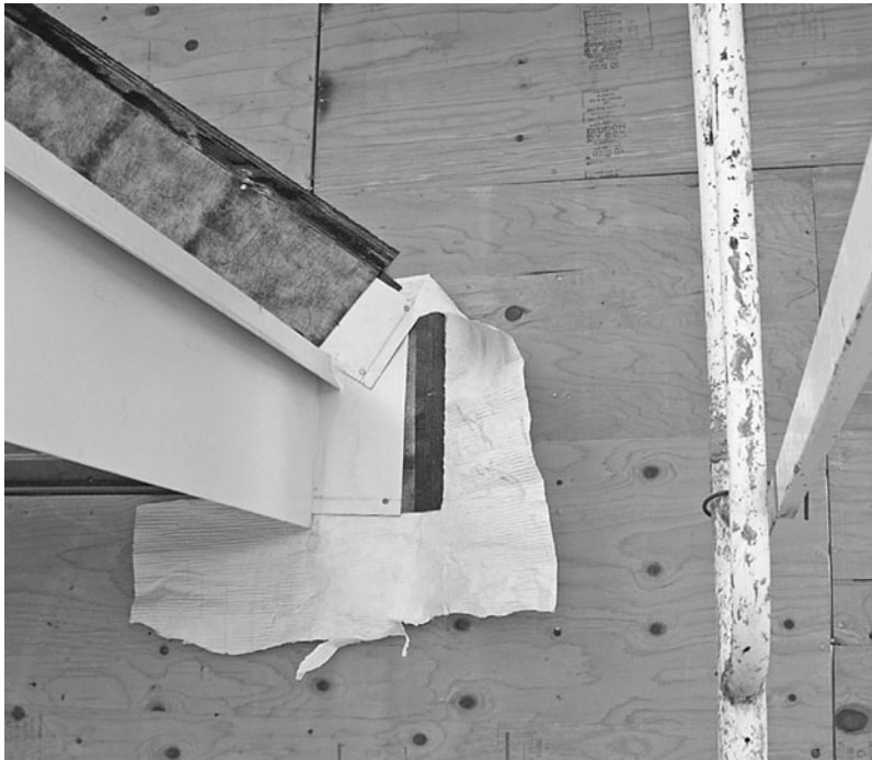
Figure 4-87 Roof to sidewall ready for membrane.
