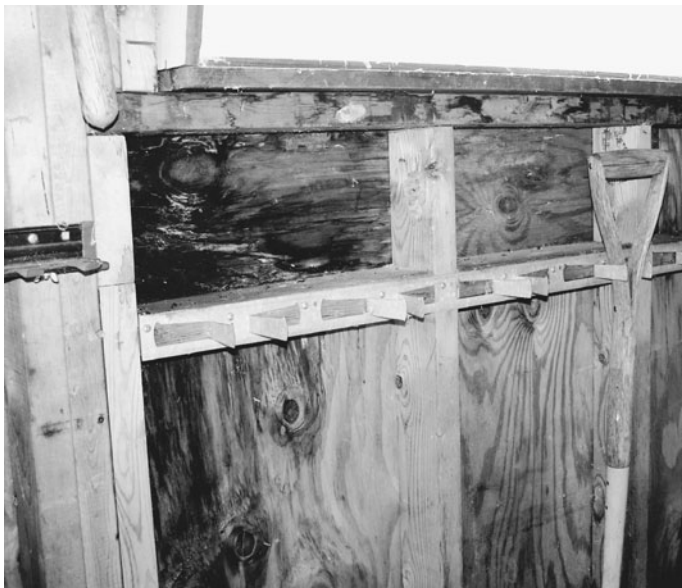
Figure 1-9 Moldy sheathing.
