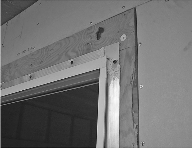
Figure 4-70 SAM window wrap, step 1.
