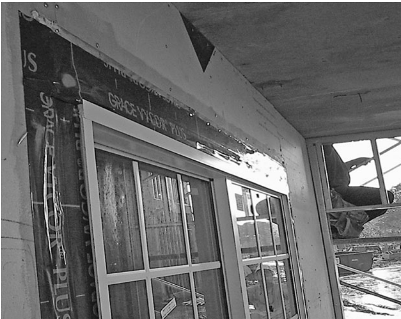
Figure 4-71 SAM window wrap, step 2.
