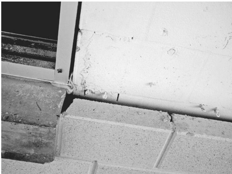
Figure 2-12 Designs should avoid reliance upon sealant.
