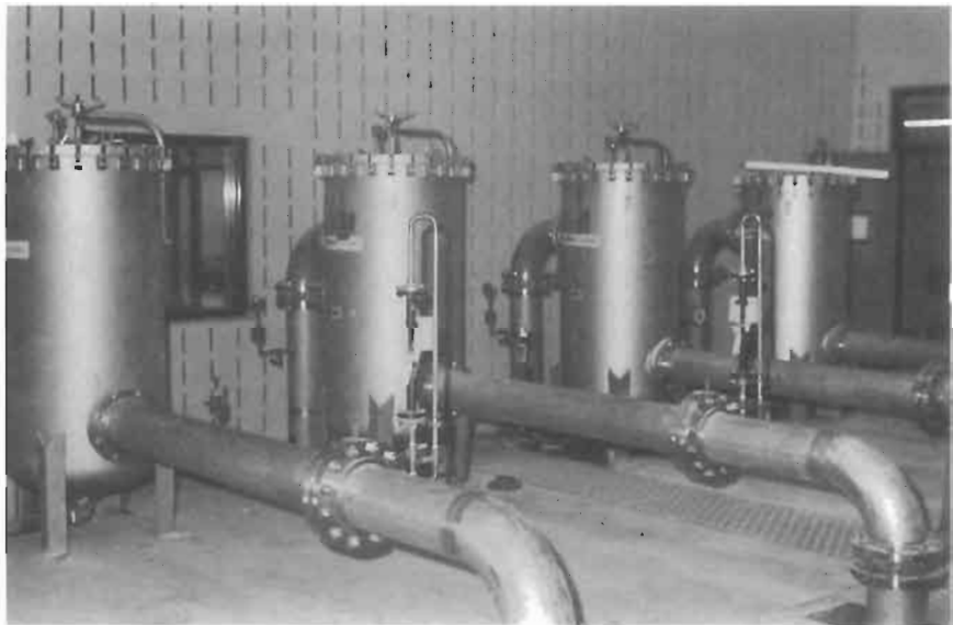
Figure 1. Battery of cartridge filters used for water pretreatment in an RO process.
