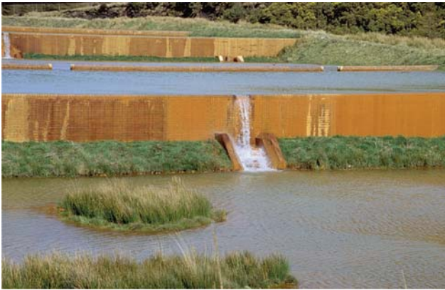
Fig. 91. Mine water overflowing the Pelenna II/Wales system. The hydraulic head is too low to drive the water through the compost (24 March 2000).
