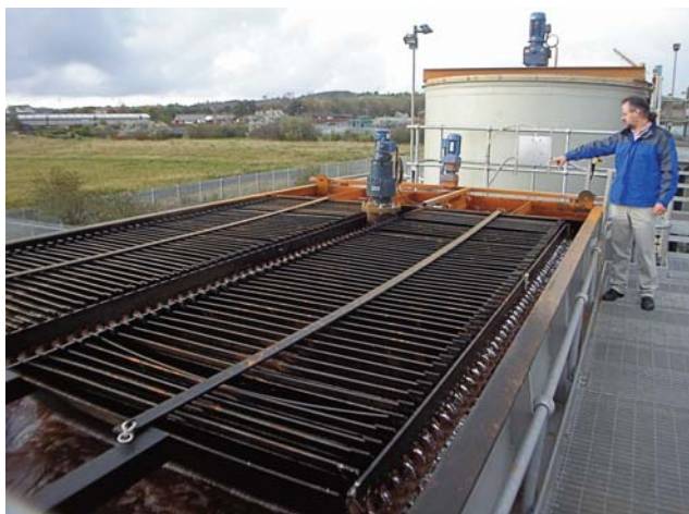
Fig. 87. Lamella clarifier at the Horden/United Kingdom HDS mine water treatment plant (photograph courtesy Andrea Berger).
