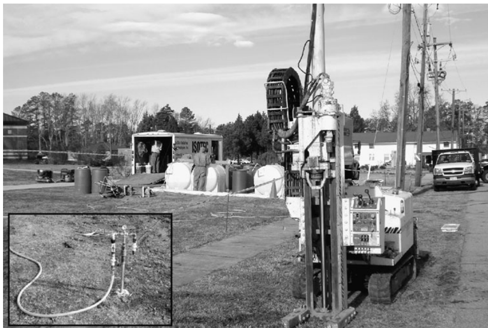
FIGURE 9.32 Direct-push drilling for oxidant injection into shallow aquifer contaminated with chlorinated solvents. Inset: Temporary injection point with the oxidant feed line. (Photographs courtesy of ECC)
