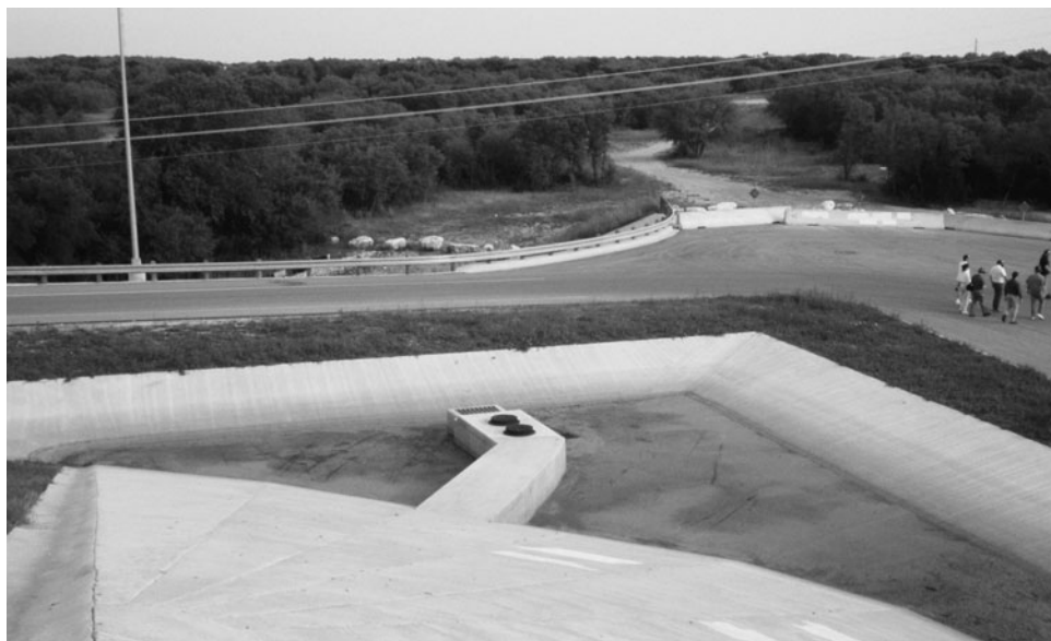
FIGURE 8.25 Concrete catch basin by a state highway in Austin, TX, designed to strip oil and fines from surface runoff before water is allowed to infiltrate into the underlying Edwards aquifer.
