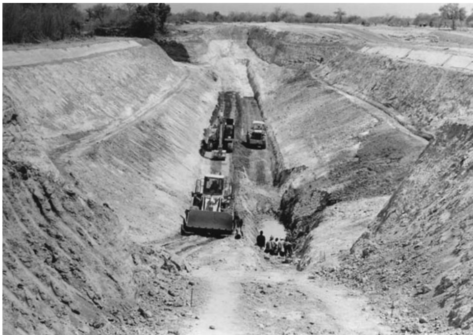
FIGURE 7.28 Construction of one of the largest subsurface earth-fill dams in Africa located in Nare Village, Burkina Faso. (From Ministry of the Environment, 2004.)
