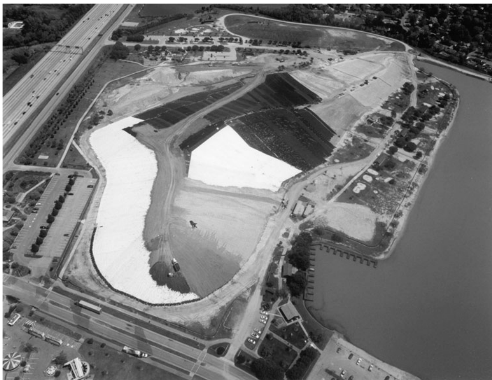
FIGURE 5.10 Aerial view of the proper closure of a modern-day landfill, which is required by strict environmental regulations. The landfill is being covered by several layers of materials to prevent rainfall infiltration and leaching, and to ensure no future adversarial impact on groundwater resources. Note the highway on the left for scale. (Printed with permission of the City of Virginia Beach, VA, the United States.)
