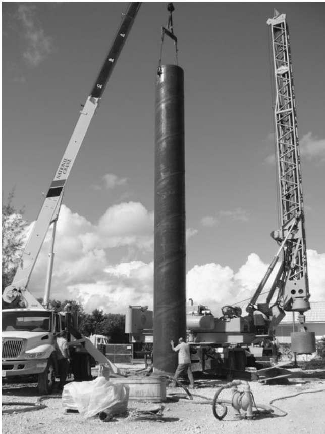
FIGURE 7.3 A 48-in.-diameter surface casing being placed in a 54-in.-diameter borehole. The target depth for the well is 1300 ft with an open interval from 1000 to 1300 ft in the Floridan aquifer. The final casing inside diameter is 20 in. The well is drilled for water supply of the city of Miramar, FL. (Photograph courtesy of Richard Crowles.)
