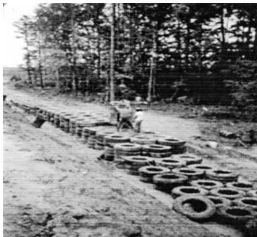
Fig. 1 Scrap tire retaining wall constructed in 1991 in Chapel Hill, North Carolina
