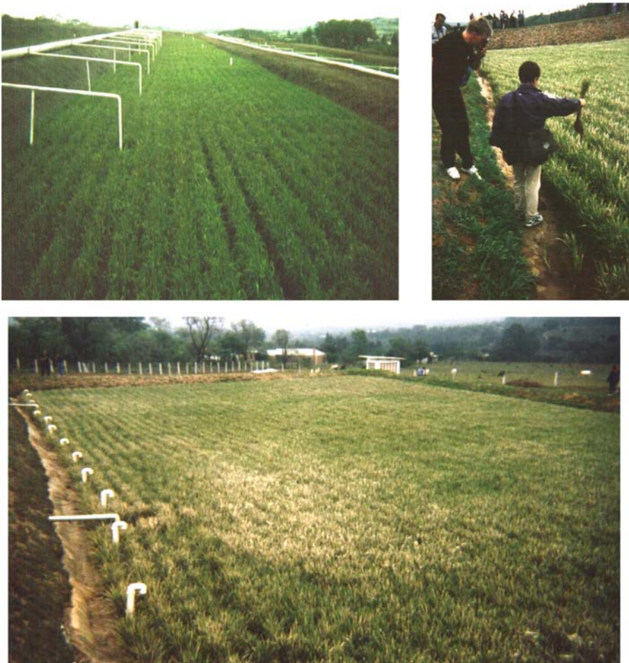
Figure 4-48. VF upflow constructed wetlands planted with rice ( Oryza sativa ) near Piracicaba, Brazil. Photos by Jan Vymazal.
