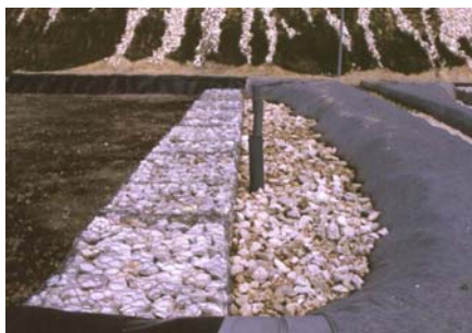
Figure 5-18. Mesh gabions in the inflow (left) and outflow (right) zones in HF constructed wetland near Leiria, Portugal. Photos by Jan Vymazal.
