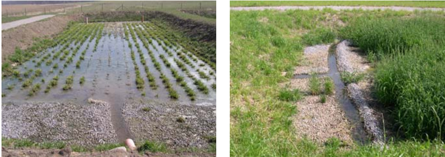
Figure 5-31. Distribution of wastewater in HF CW Břehov, Czech Republic. Left: Wastewater flows through the middle of the bed causing shortcircuiting, right: raised wall which spreads the wastewater along the whole inlet zone. Photos by Lenka Kröpfelová.
