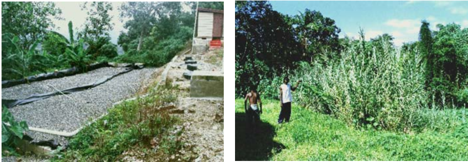
Figure 7-43. HF constructed wetlands at Pishah (left, before planting) and Retrive (right, planted with wild cane, Gynerium sagittatum ) in Jamaica. Photos by Ed Stewart, with permission.
