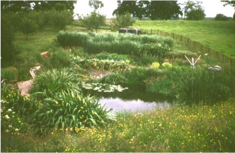
Figure 4-42. Hybrid system at Oaklands Park, UK. The first VF stage ( 6 \times 8 \text{ m}^2 ) is composed of six beds planted with Phragmites australis (top back of the picture), the second VF stage (below, 3 \times 5 \text{ m}^2 ) is composed of three beds planted with Scirpus lacustris , Iris pseudacorus and P. australis . The third HF stage ( 8 \text{ m}^2 ) is planted with I. pseudacorus and the 4 th HF stage ( 20 \text{ m}^2 ) is planted with Acorus calamus , S. lacustris , Carex elata and Sparganium erectum . Photo by Jan Vymazal.
