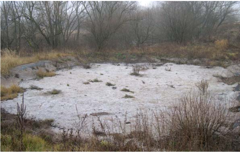
Figure 7-21. HF constructed wetland at Náplepkovo, East Slovakia (500 m 2 ) designed for tertiary treatment of dairy wastewaters. The system built in 1992 is currently out of operation because the dairy was closed down. Photo by Jan Vymazal.
