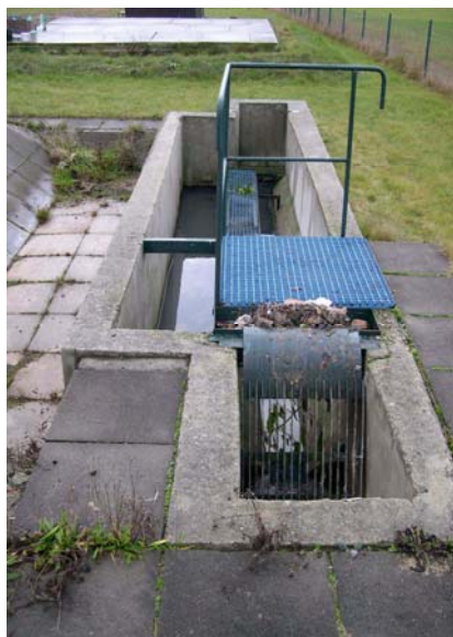
Figure 5-10. Left: grit chamber after the bar screens (CW Slavošovice, Czech Republic, photo by Lenka Kröpfelová), right: grit chamber preceding the screens (CW Kámen, Czech Republic, photo by Jan Vymazal).
