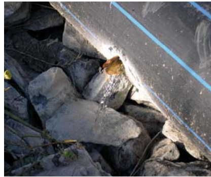
Figure 5-27. Distribution pipes on the surface of distribution zone. HF CW Čehovice, Czech Republic. Left: general view, right: detail of the wastewater inflow. Photos by Lenka Kröpfelová.
