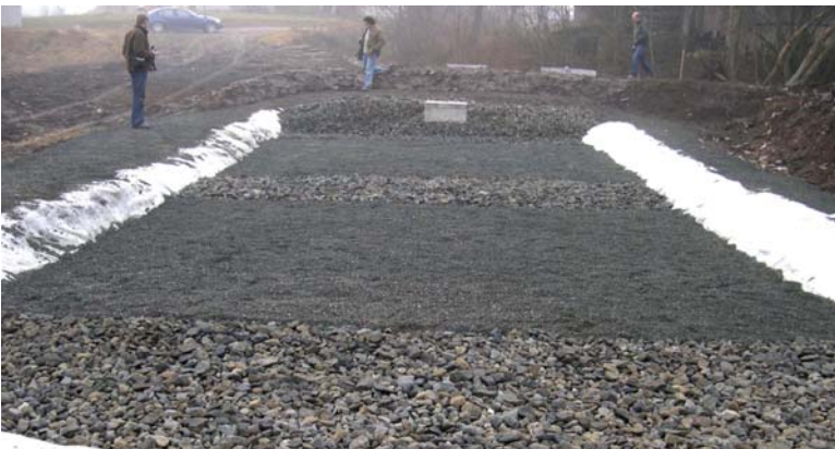
Figure 7-22. HF constructed wetland for secondary treatment of municipal sewage at Zadný Hámor, East Slovakia (17 PE, 90 m 2 ) after completion in November 2006. Photo by Jan Vymazal.
