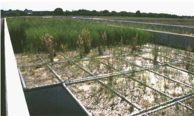
Figure 4-38. FWS constructed wetland with floating rafts with Phragmites australis at London Heathrow International Airport treatment system. Photo by Jan Vymazal.
