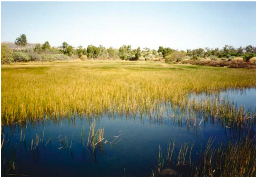
Figure 4-32. FWS constructed wetland planted with Eleocharis dulcis for the treatment of mine waters from Ranger uranium mine at Jabiru, Northern Territory, Australia. Photo by David Jones, with permission.
