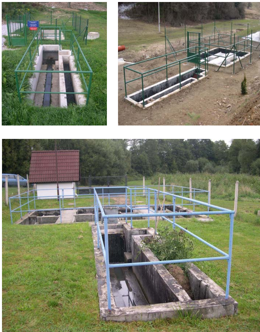
Figure 5-15. Examples of pretreatment for secondary treatment HF constructed wetlands for 100 PE (top left, Petrovice, Czech Republic), 200 PE (top right, Skuhrov, Czech Republic) and 500 PE (bottom, Dolní Město, Czech Republic). All systems consist of screens, horizontal grit chamber and Imhoff tank. Photos by Lenka Kröpfelová.
