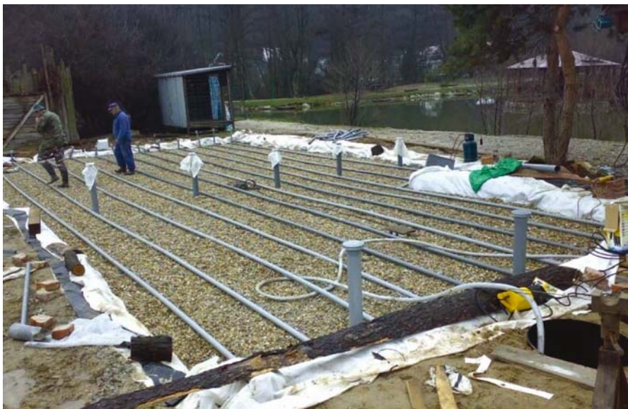
Figure 4-46. Distribution of wastewater across the surface of VF bed at Bojna, Slovakia. Photo by Milan Raffesberg, with permission.
