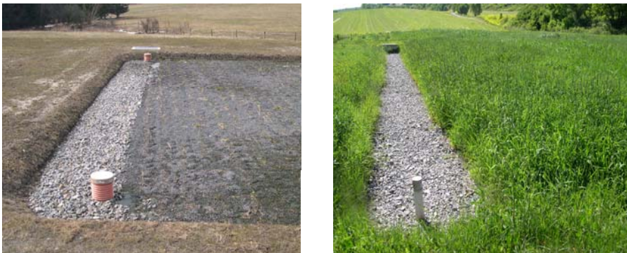
Figure 5-32. Outflow zones are leveled with the filtration bed surface. The zones are frequently equipped with inspection pipes. Left: CW Sklené, Czech Republic, right: CW Mořina, Czech Republic. Photos by Jan Vymazal.
