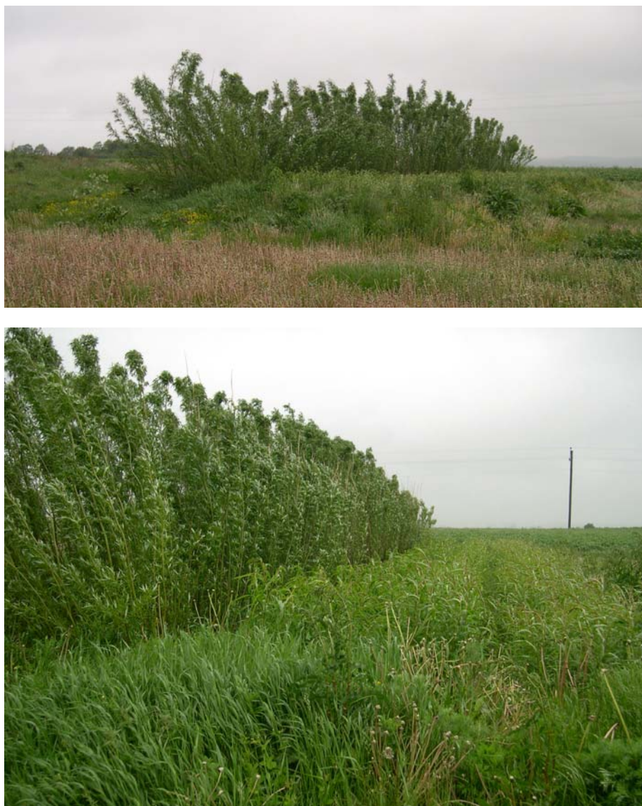
Figure 4-60. Willow based constructed wetland at Vråvej, Denmark. One third of aboveground biomass is harvested every year. Photos by Jan Vymazal.
