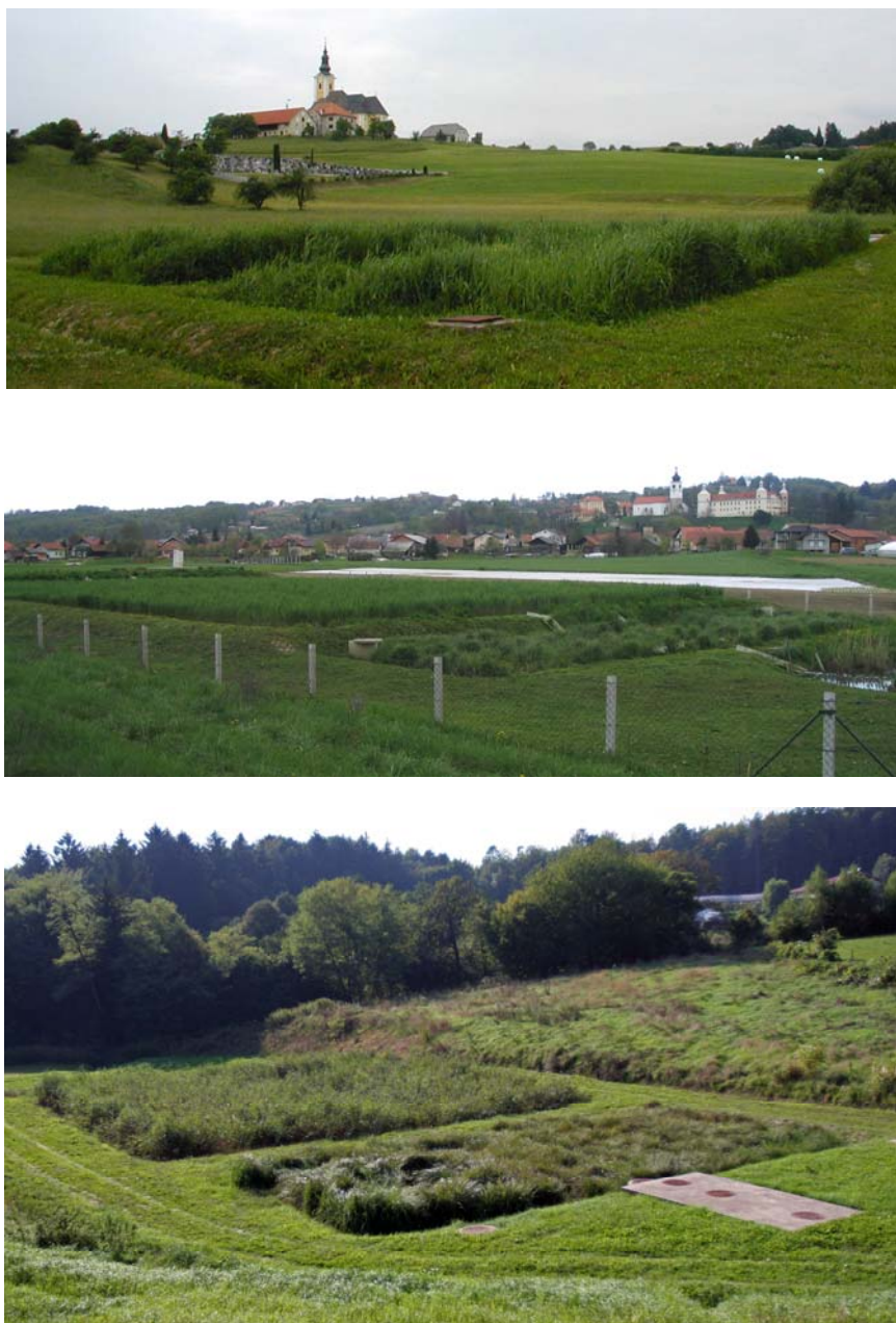
Figure 7-24. HF constructed wetlands for municipal sewage in Slovenia. Top: Ponikva, a 600 m 2 system built in 1992 (photo by Tjaša Griessler Bulc, with permission); middle: Velika Nedelja, a hybrid system consisting of HF bed (100 m 2 ), two VF beds (350 m 2 each), HF bed (100 m 2 ) and FWS pond (64 m 2 ) built in 2000 for 400 PE (photo by Tjaša Griessler Bulc, with permission); bottom: Sveti Tomaž, a 700 m 2 HF system with four beds for 250 PE built in 2001 (photo by Bogdan Macarol, with permission).
