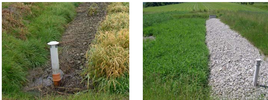
Figure 5-29. Inspection pipes at the end of inflow zone. Left: CW Čejkovice, right: Mořina, Czech Republic. Photos by Jan Vymazal.
