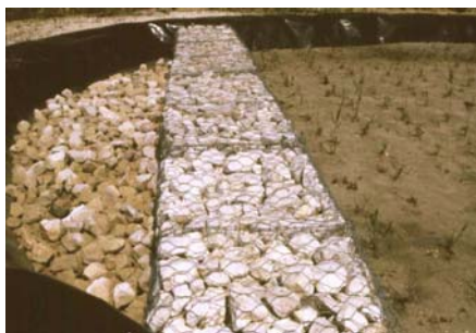
Figure 5-18. Mesh gabions in the inflow (left) and outflow (right) zones in HF constructed wetland near Leiria, Portugal. Photos by Jan Vymazal.
