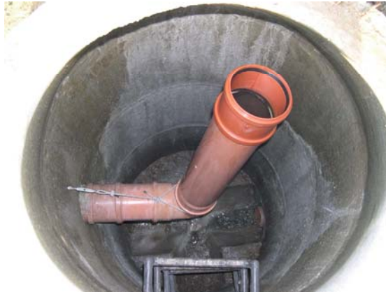
Figure 5-33. Socketted pipe at the outflow from a HF CW in Krásna Lúka, Slovakia, Photo by Jan Vymazal.
