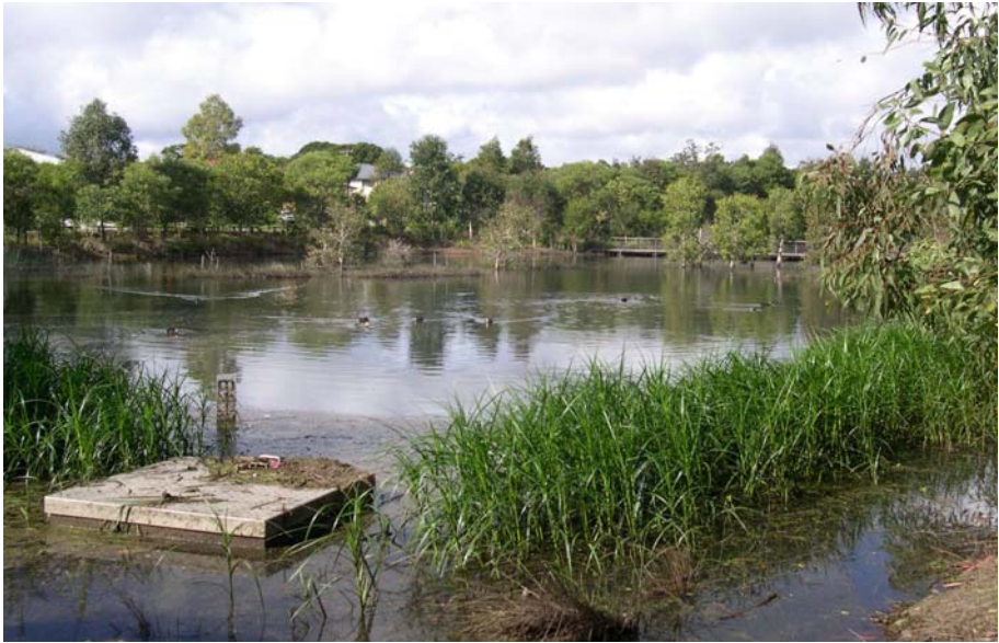
Figure 4-20. Outflow structure in a stormwater treatment constructed wetland, Brisbane, NSW, Australia. Photo by Jan Vymazal.
