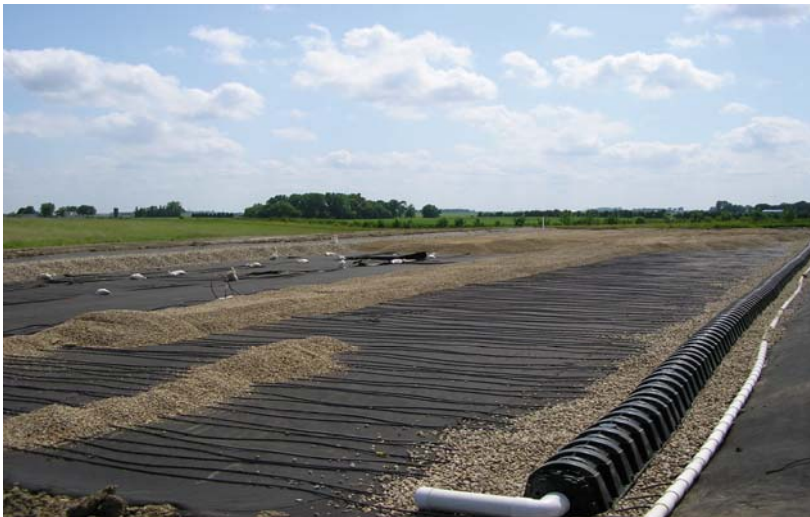
Figure 7-36. Installation of influent distribution chamber and aeration lines for HF CW at Prinsburg, Minnesota, U.S.A. Photo by Scott Wallace, with permission.
