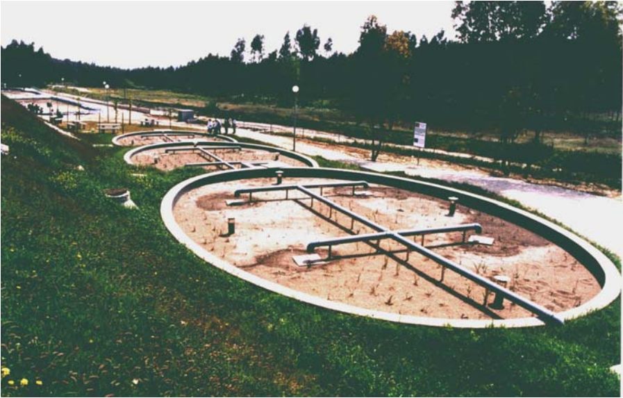
Figure 4-45. Wastewater distribution at vertical flow constructed wetland which is a part of the treatment system for landfill leachate near Leiria, Portugal. Photo by Jan Vymazal.
