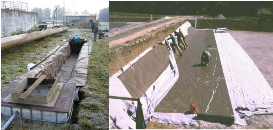
Figure 5-16. Left: plastic liner at the experimental HF constructed wetland at Třeboň, Czech Republic. Right: Plastic liner in between two layers of geotextile (CW Mořina, Czech Republic). Photos by Jan Vymazal.
