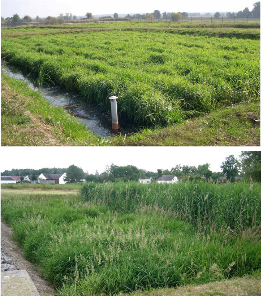
Figure 5-46. Top: HF constructed wetland Čejkovice, Czech Republic planted with Phalaris arundinacea as single species. Bottom: HF constructed wetland Příbraz, Czech Republic planted with Phalaris arundinacea (at left) and Phragmites australis in bands perpendicular to flow path. Photos by Lenka Kröpfelová.
