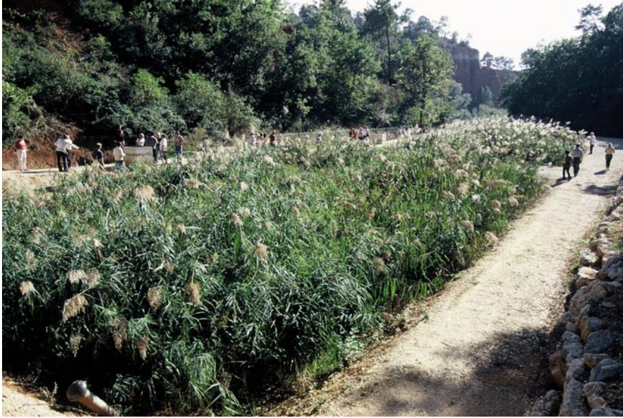
Figure 4-44. VF constructed wetlands treating raw sewage from 1,200 PE in Roussillon, France. Photo by Jan Vymazal.
