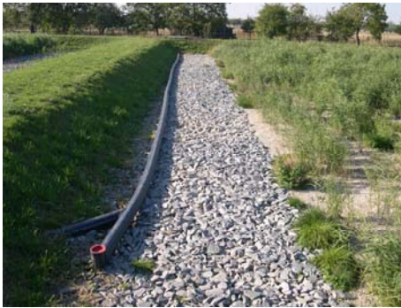
Figure 5-27. Distribution pipes on the surface of distribution zone. HF CW Čehovice, Czech Republic. Left: general view, right: detail of the wastewater inflow. Photos by Lenka Kröpfelová.
