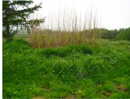
Figure 4-43. A single bed VF constructed wetland ( 15 \text{ m}^2 ) at Mørke, Denmark, planted with Phragmites australis . Left: shortly after planting in 2002 (from Arias and Brix, 2005a, with permission from Backhuys Publishers), Right: in June 2005, photo by Jan Vymazal.
