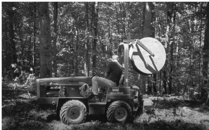
Photo 5.5b Drip system for effluent dispersal installed in wooded area using a vibratory plow.
