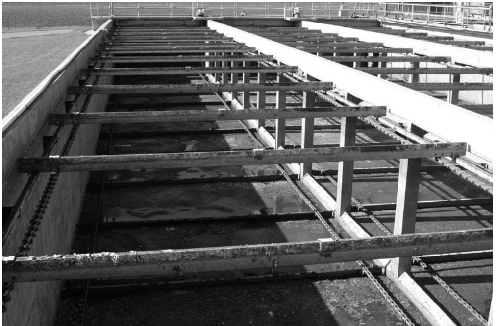
FIGURE 9.7 An example of a rectangular sedimentation tank.
