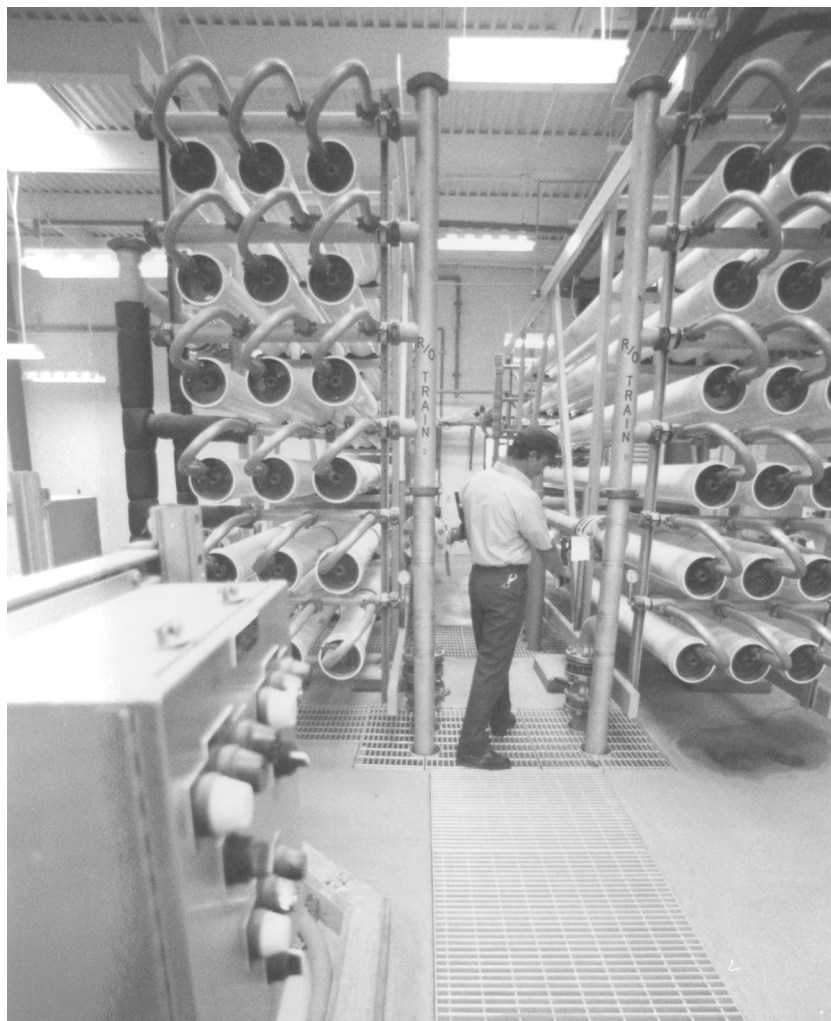
Checking the reverse osmosis unit at San Diego's Aqua III water reclamation facility. Photo by Joe Klein.
