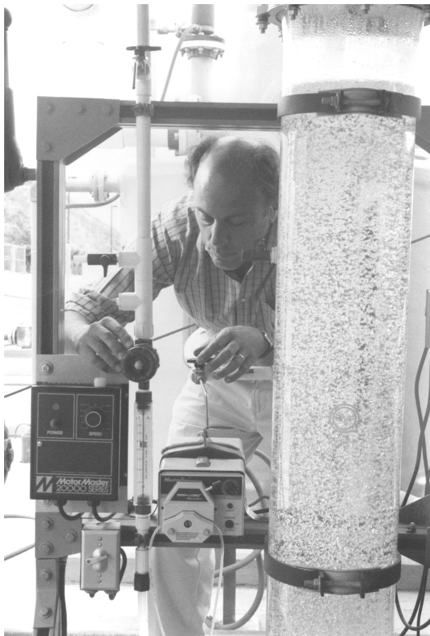
Checking the ozone disinfection unit at San Diego's Aqua III water reclamation facility. Photo by Joe Klein.
