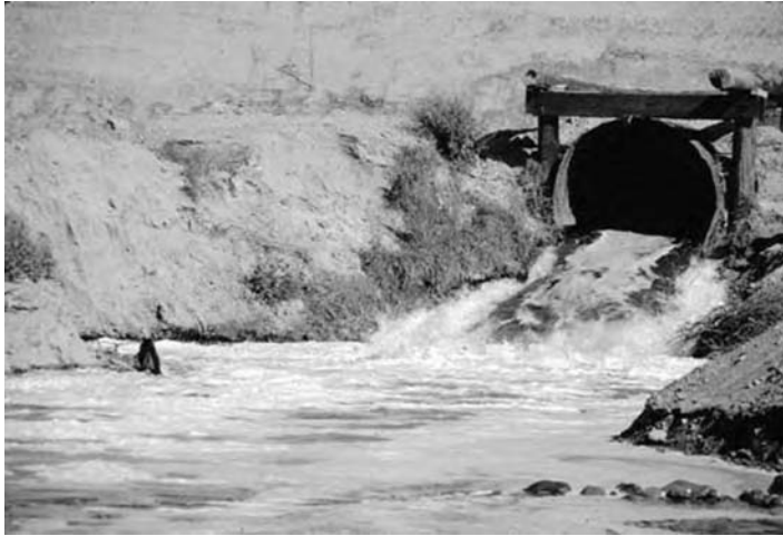
FIGURE 9.4 Outfall pipe. (From University of Arizona, 2005 Photo by Barbara Tellman.)
