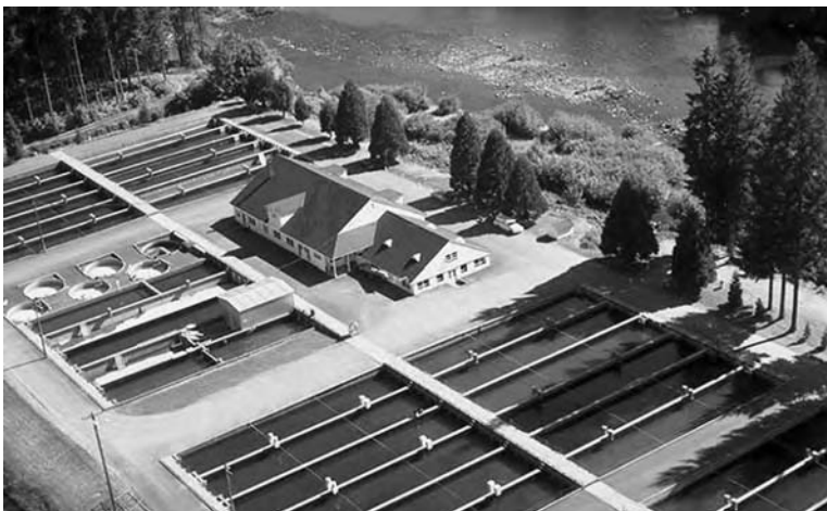
FIGURE 4.16 Fish hatchery on the Columbia River. (From USACE, 2005e.)
