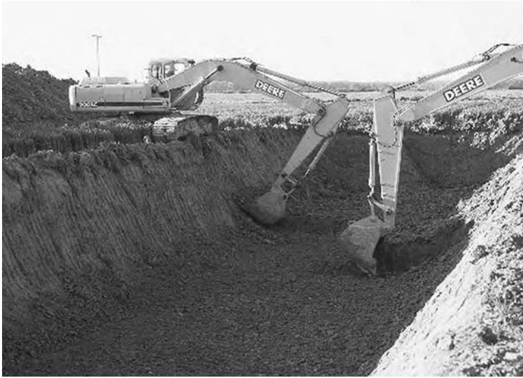
FIGURE 9.49 Tailwater pit. (From NRCS, 2005e.)
