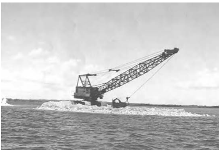
FIGURE 6.13 Dredge-and-fill operation. (From USGS, 2005g.)
