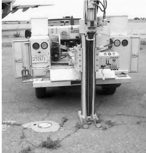
FIGURE 7.14 Soil-gas probe. (From USACE, 2005c.)
