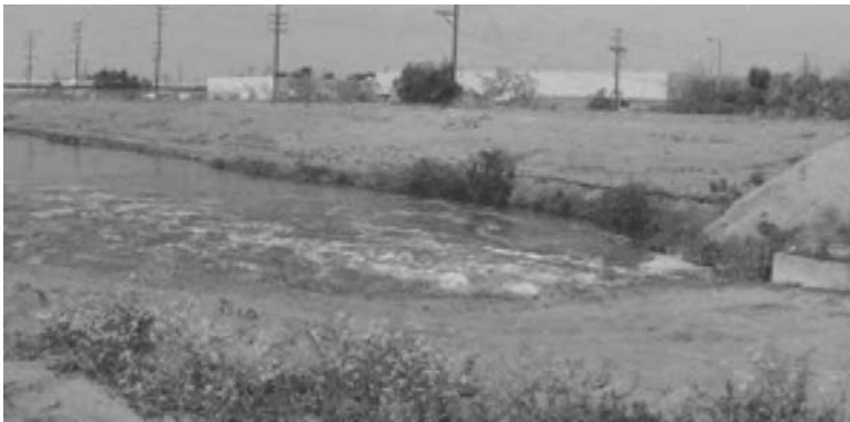
FIGURE 7.4 Wastewater infiltration basin. (From NEWater, 2005.)
