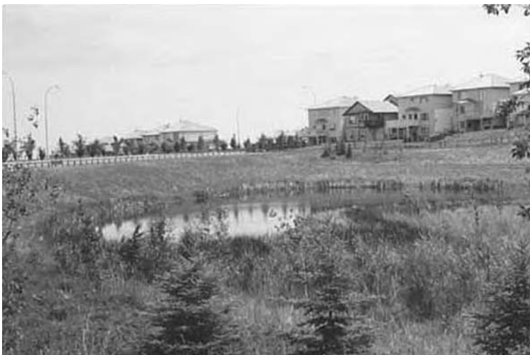
FIGURE 9.24 Constructed wetland for stormwater runoff. (From Bow River Basin Council, 2005.)
