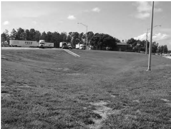
FIGURE 9.14 Infiltration basin. (Courtesy of David A. Chin.)
