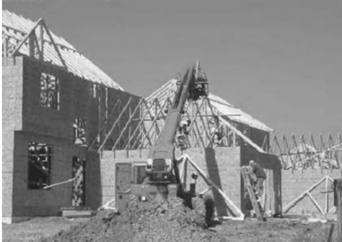
FIGURE 9.8 Typical residential construction site.
