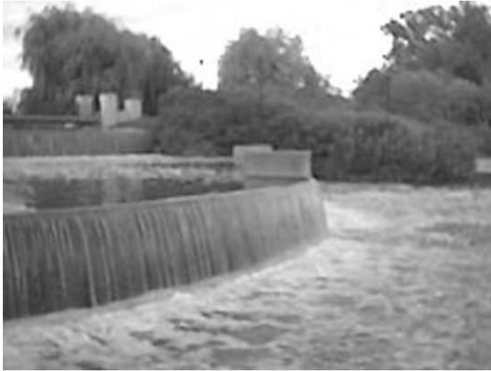
FIGURE 4.19 Sidestream aeration in Worth, Illinois. (From Chicago Public Library, 2005.)
