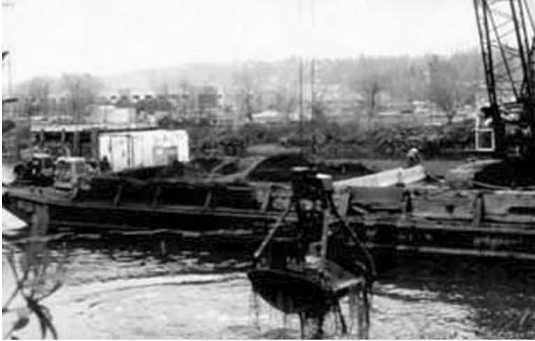
FIGURE 4.22 Dredging of contaminated sediment. (From Seattle Daily Journal of Commerce , 2005.)
