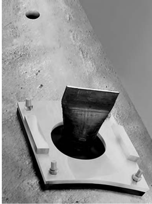
FIGURE 8.9 Diffuser ports. (Courtesy of Philip J. W. Roberts.)
