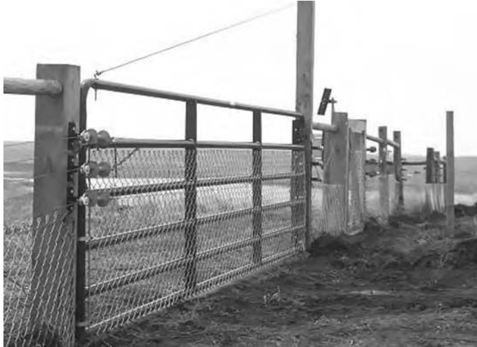
FIGURE 6.20 Fence for wildlife exclusion. (From U.S. Fish and Wildlife Service, 2005b.)
