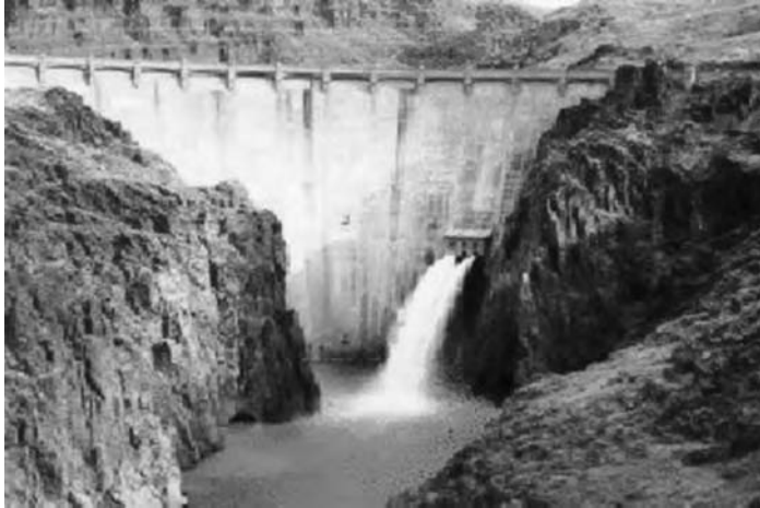
FIGURE 5.10 Low-level discharge from a lake.
