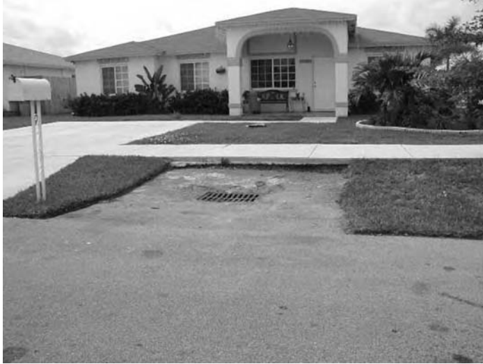
FIGURE 9.13 Direct connection between a roadway and a stormwater inlet. (Courtesy of David A. Chin.)
