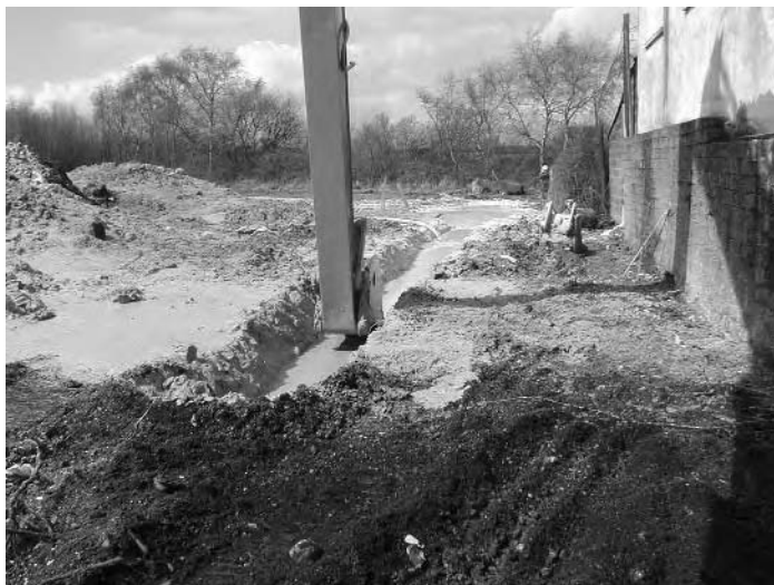
FIGURE 7.35 Construction of a slurry wall. (From Permeable Reactive Barrier Network, 2005.)
