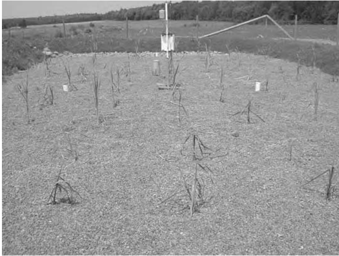
FIGURE 6.12 Constructed subsurface-flow wetland. (From Nova Scotia Agricultural College, 2005. Photo by Steven Tattreie.)
