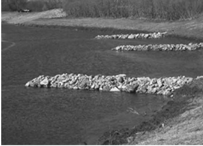
FIGURE 4.2 Deflection bars on the Little Blue River, Kansas. (From NRCS, 2005b.)
