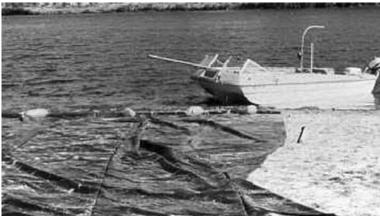
FIGURE 5.17 Application of sediment cover and lake shading. (From State of Washington, 2005.)
