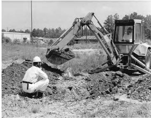
FIGURE 7.24 Soil excavation at a Superfund site. (From USACE 2005d.)
