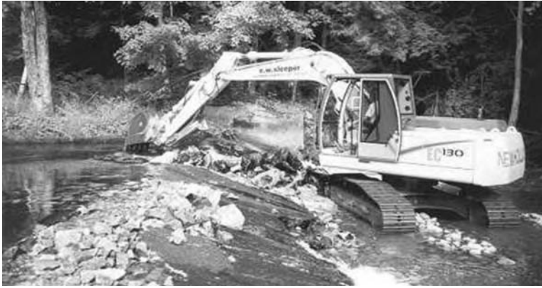
FIGURE 4.21 Dam removal on the Ashuelot River, New Hampshire. (From U.S. Fish and Wildlife Service, 2005a.)
