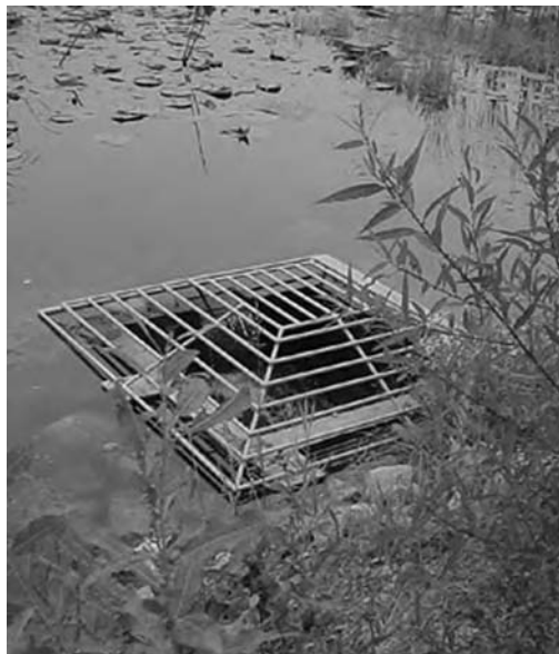
FIGURE 6.15 Wetland outlet weir. (From Emmons and Oliver Resources, 2005).
