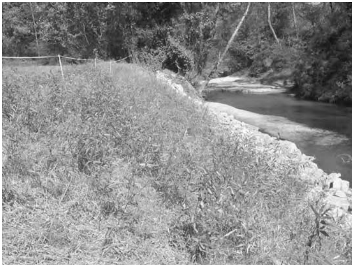
FIGURE 9.50 Stabilized channel banks. (From NRCS, 2005f.)
