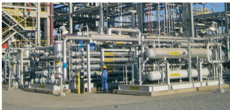
Figure 8.14 Flow diagram showing the use of hydrocarbon-permeable membranes to recover unreacted monomers from a polyolefin plant resin degassing unit. The photograph is of a system installed by MTR in Qatar in 2007.
