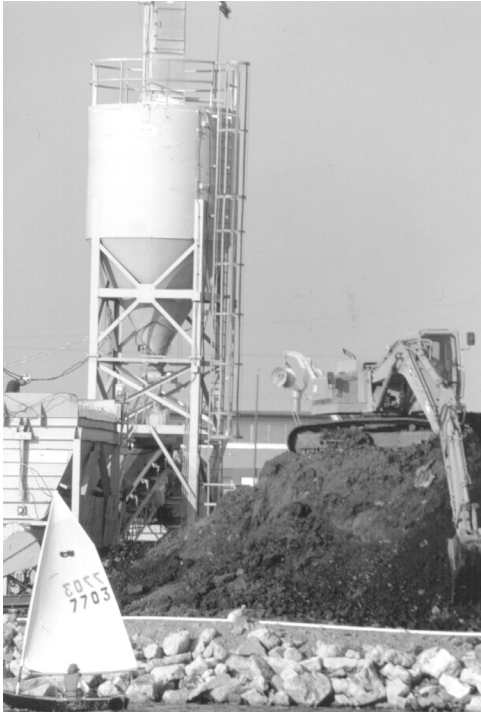
A former fuel storage and handling facility in California was demolished to make way for a marina. As part of the process, 13,000 m 3 of petroleum-contaminated soils were treated in above-ground bioremediation cells. Courtesy of Fluor Daniel GTI.
