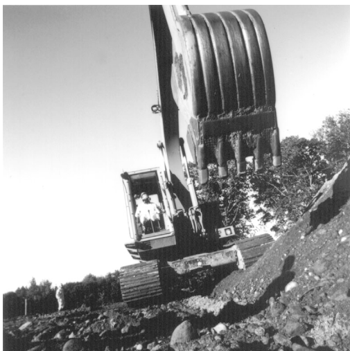
Excavation of soil at a contaminated site. Courtesy of Fluor Daniel GTI.
