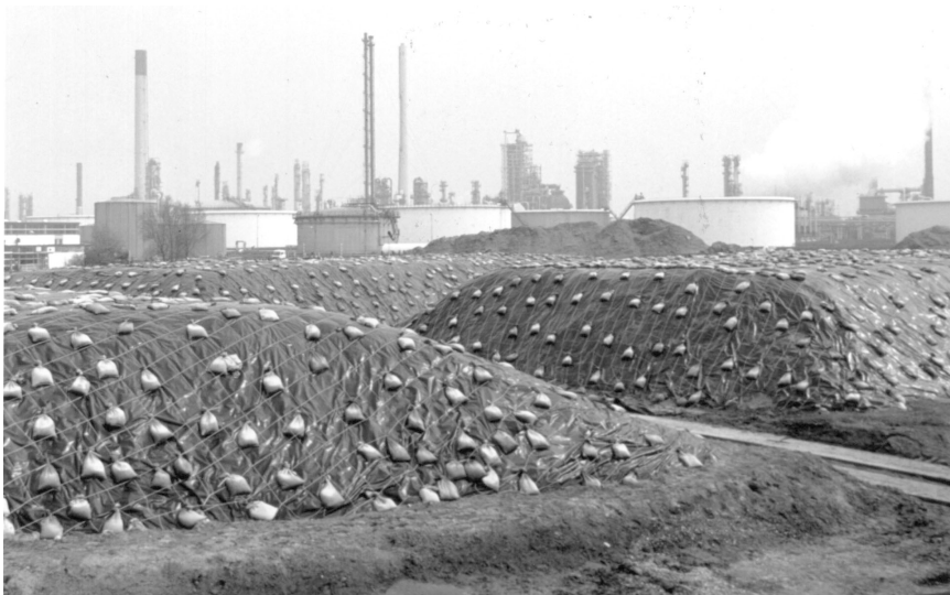
Petroleum-contaminated soils being treated in above-ground bioremediation cells engineered with vapor extraction systems. Courtesy of Fluor Daniel GTI.
