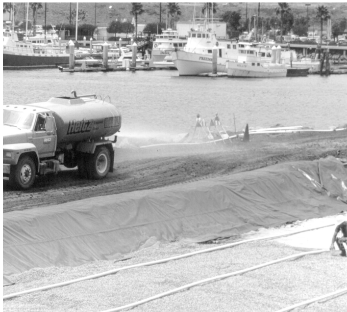
In above-ground bioremediation cells (under construction), oxygen is supplied to soil via a network of embedded piping. Courtesy of Fluor Daniel GTI.
