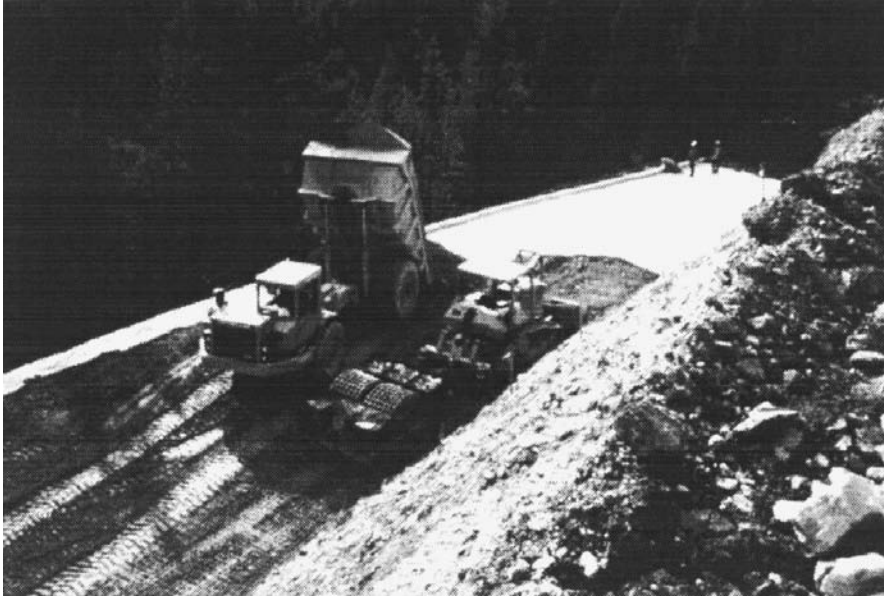
FIGURE 27.6 Placement of a high-strength nonwoven geotextile to perform a dual function of reinforcement and in-plane drainage in a reinforced slope.
