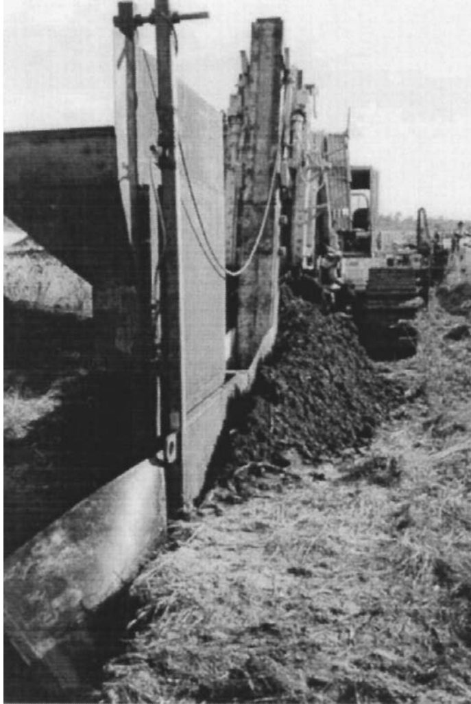
FIGURE 27.18 One pass trencher for installation of an HDPE vertical barrier system. (Photo courtesy of Groundwater Control, Inc.)
