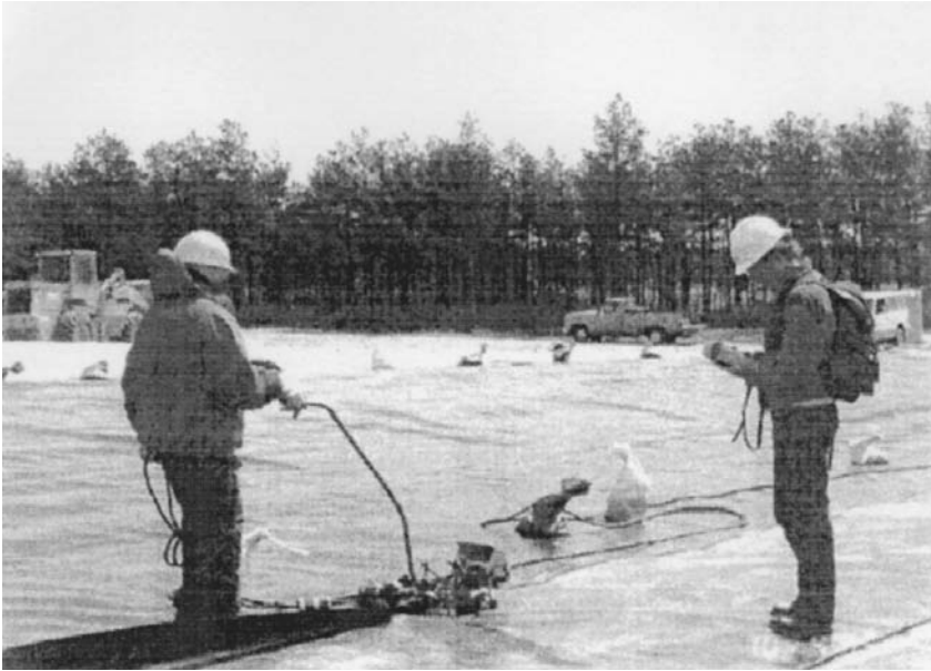
FIGURE 27.9 Monitoring seaming of a geomembrane liner.
