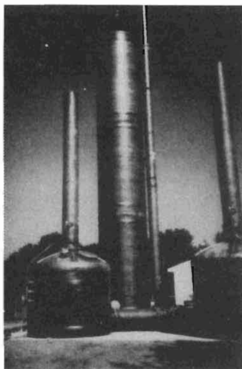
Fiberglass-reinforced plastic packed column with two carbon vapor phase treatment units; Battle Creek, MI.
