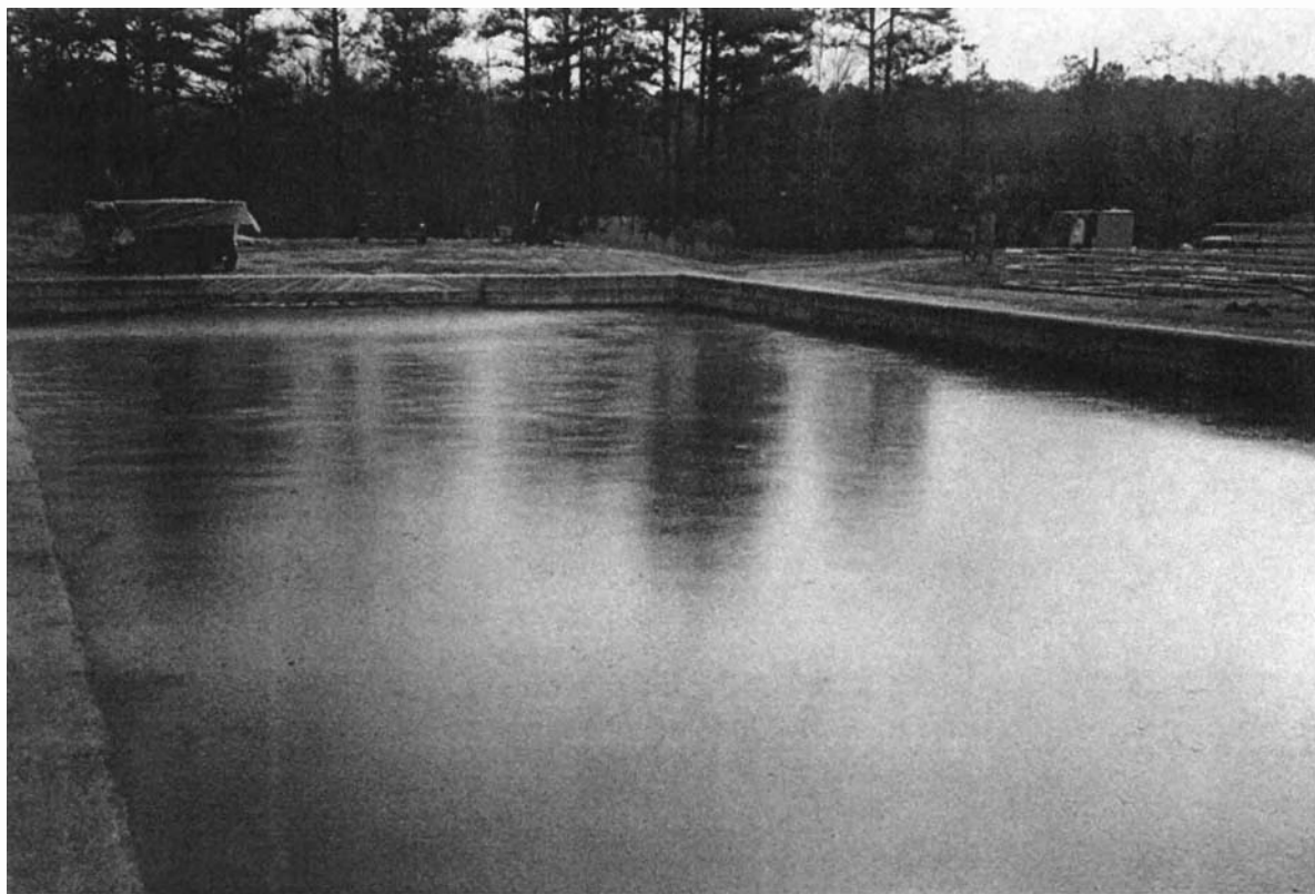
Photo 24.4a Sludge drying bed.
