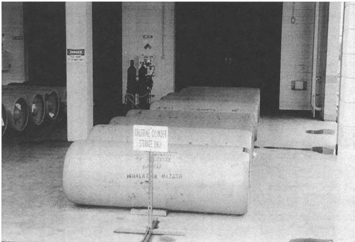
Photo 8.1 One ton chlorine tanks.
