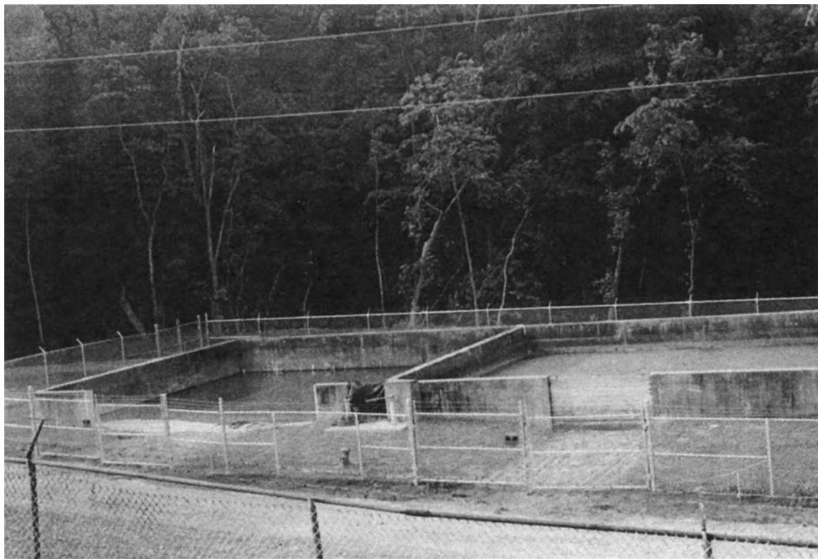
Photo 22.1 Alum sludge drying beds, left side empty, right side full.
