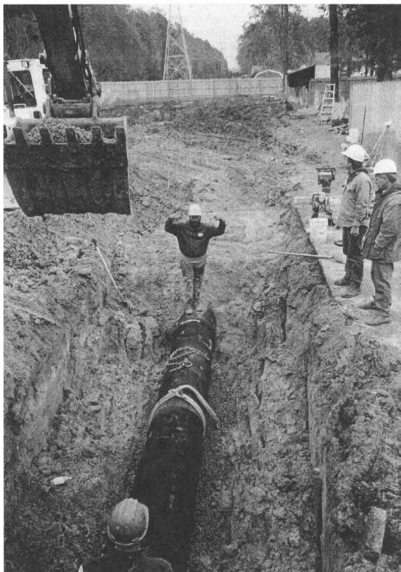
Photo 13.4b Replacing interceptor pipe.
