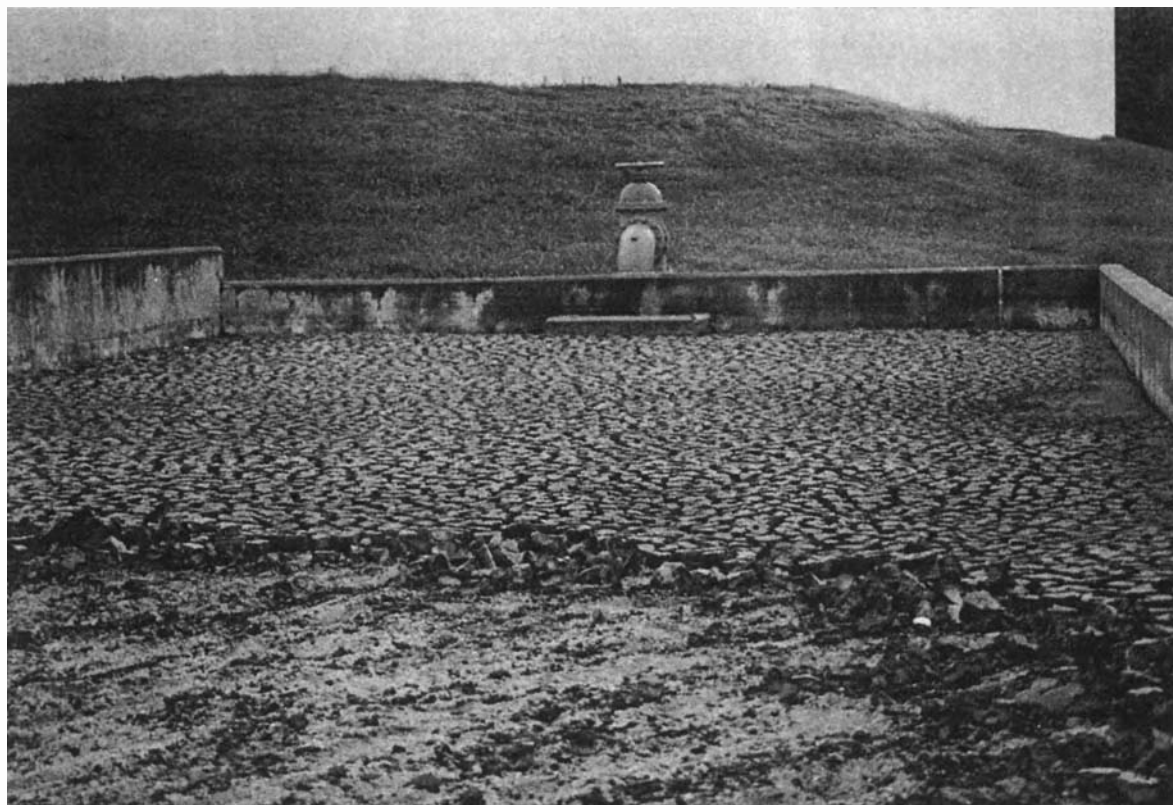
Photo 24.4d Sludge drying bed (process finished).
