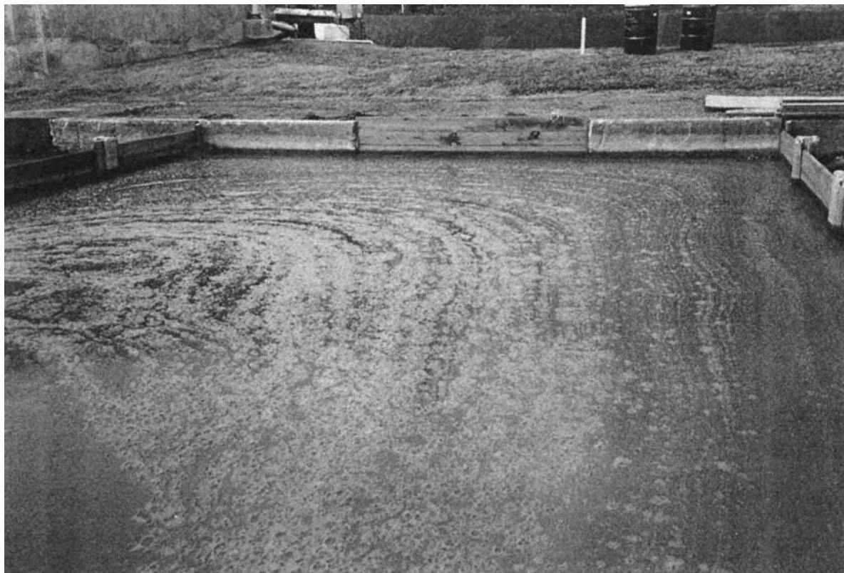
Photo 24.4b Sludge drying bed (drying in progress).
