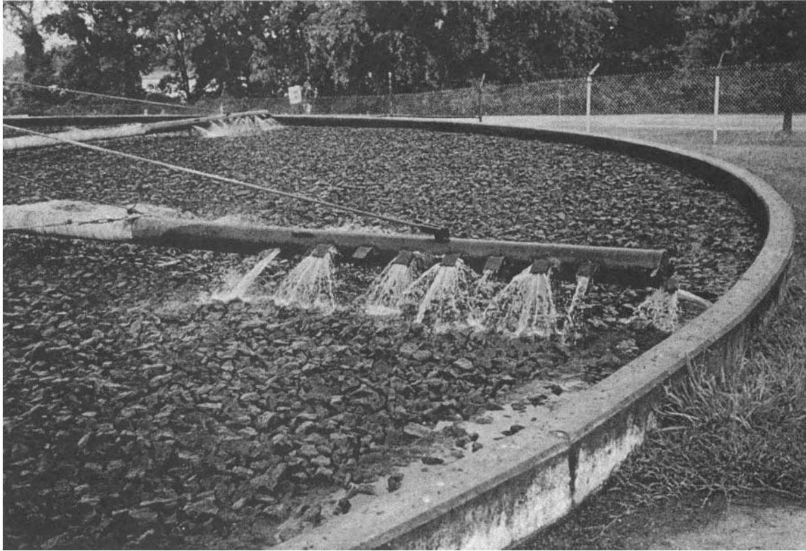
Photo 16.3 Trickling filter.
