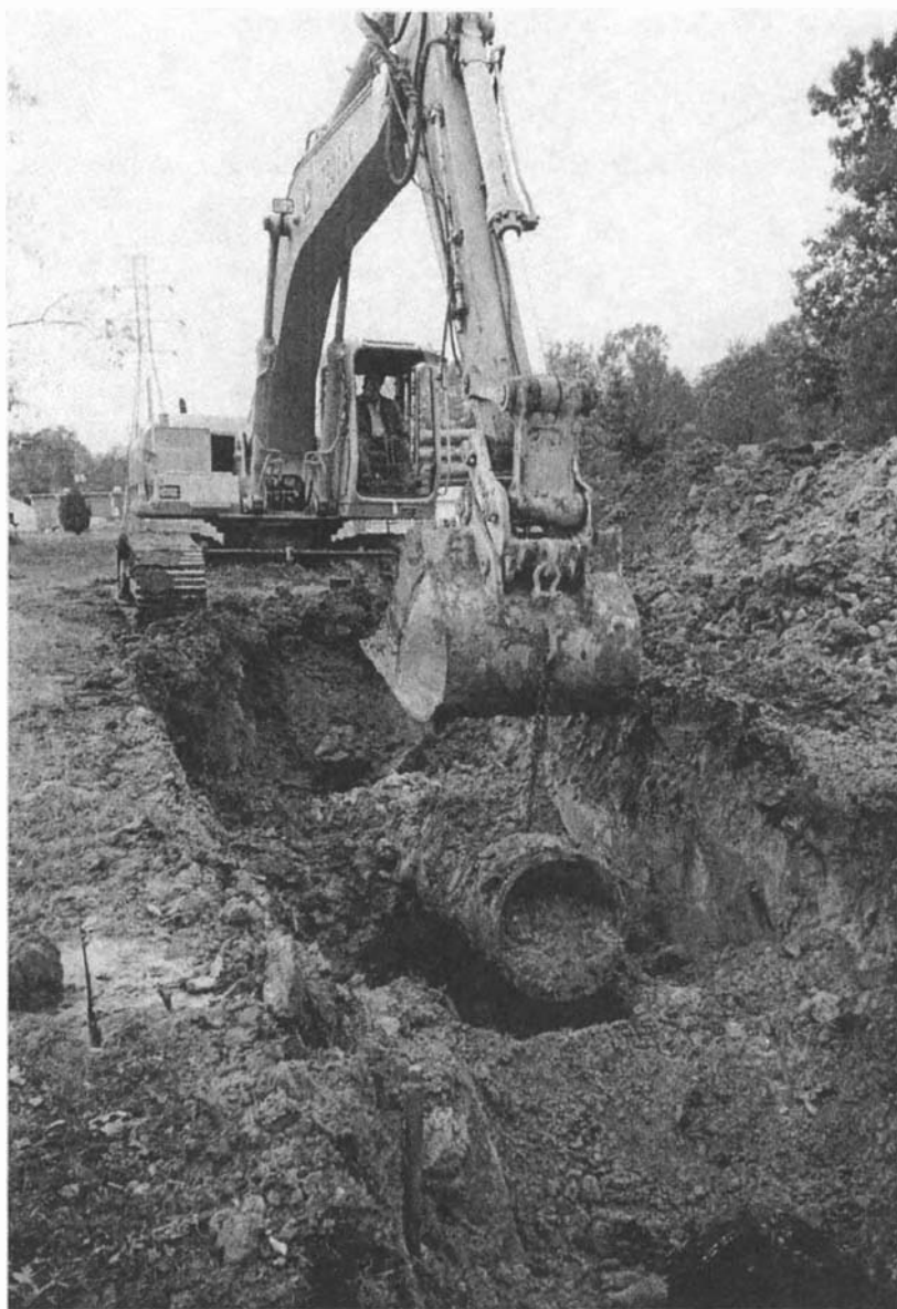
Photo 13.4a Removing broken interceptor pipe.
