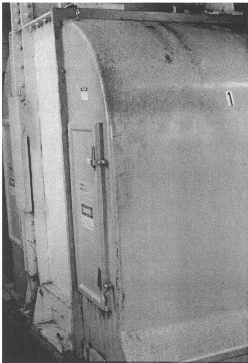
Photo 4.6 Traveling screen housing.
