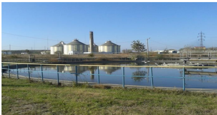
Figure 1 – WWTP anaerobic digesters studied
