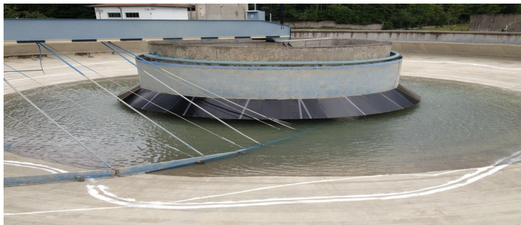
Fig. 8 – Prelungire manta deflector –decantor radial
