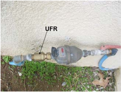
Figure 10. UFR installation
