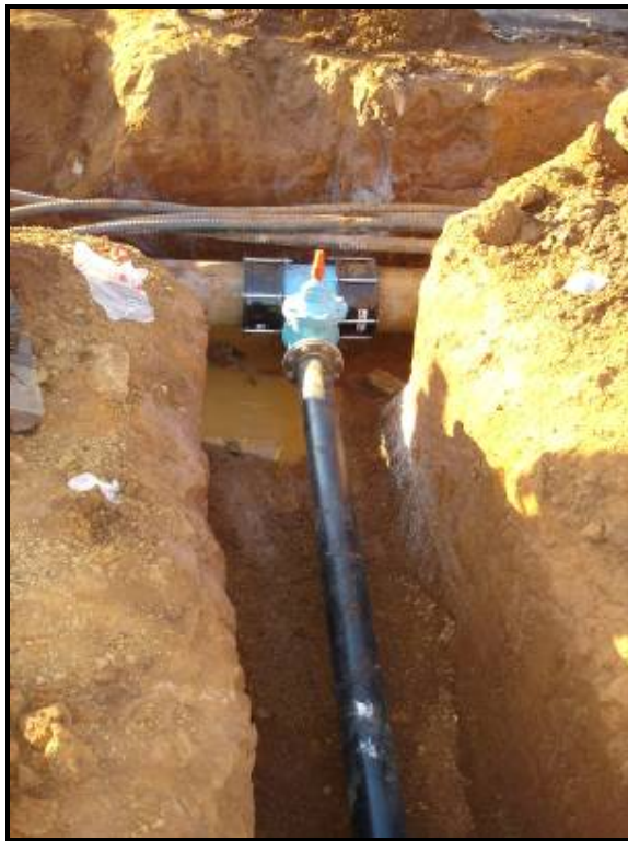
Figure 5: Installation of missing "T-Piece "in Sebokeng
