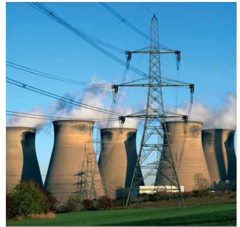
Centrale electrice Electrical power plant Kraftwerke
