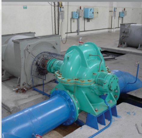
Stații de pompare Pumping Stations Pumpwerke
