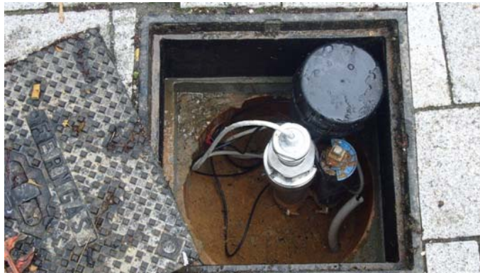
Figure 2: Built-in sluice gate
