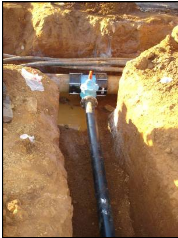
Figure 5: Installation of missing "T-Piece "in Sebokeng
