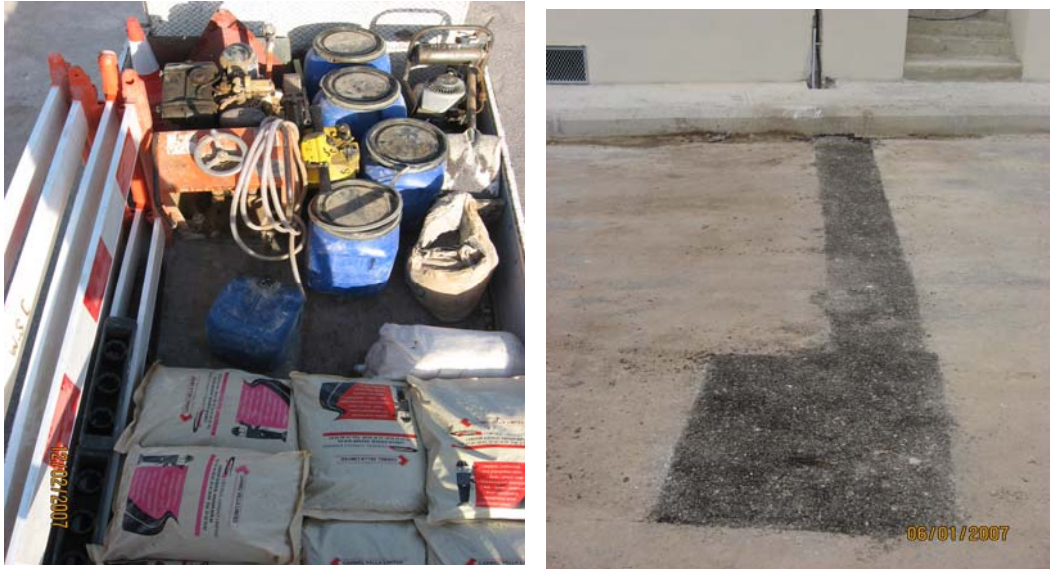
Figure 5: Truck loaded with equipment and materials for reinstatement (left) and a first attempt, new service at Marsascale (right)
