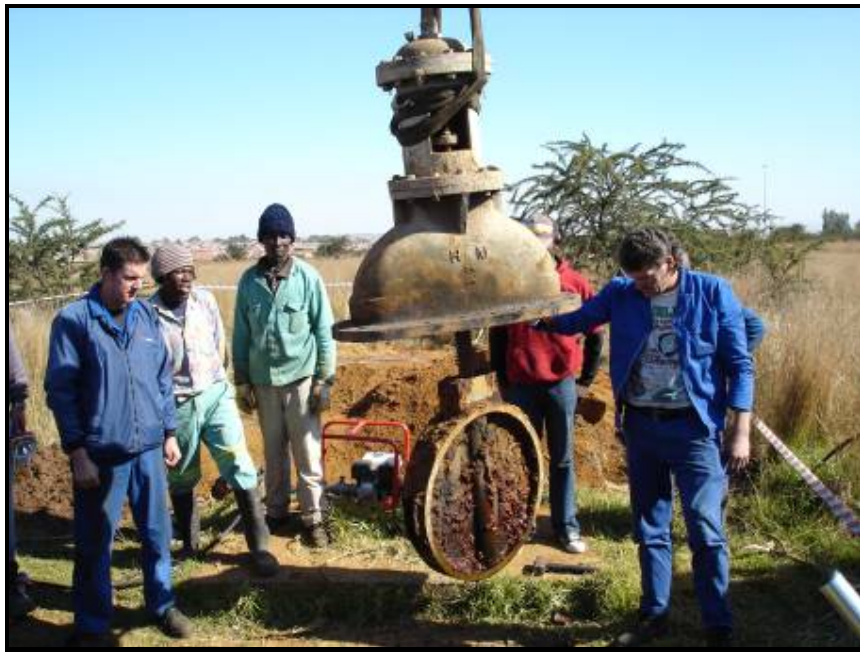
Figure 7: Removal of valve body
