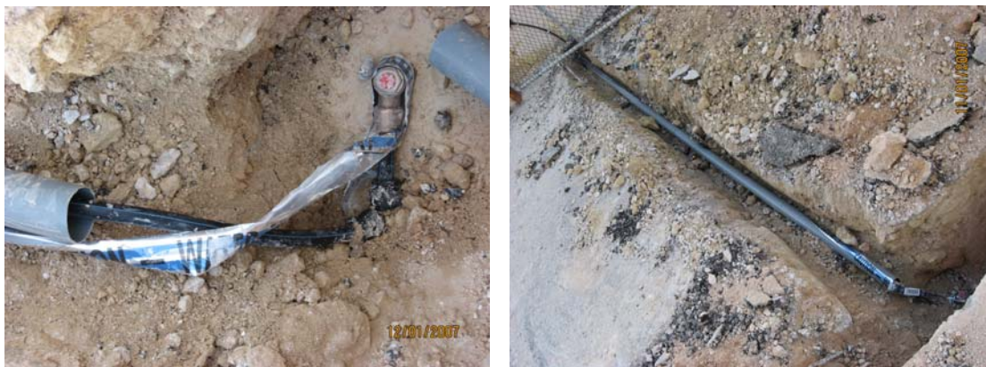
Figure 4: Tapping area with bend and start of sleeve (left) and sleeve from tapping area towards pavement
