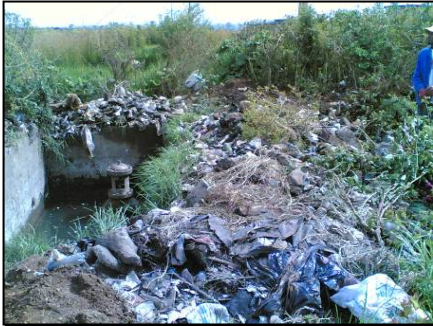
Figure 6: Identification of missing valve and chamber after cleaning
