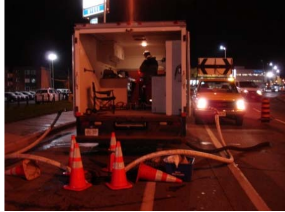
Figure 2: Above ground water supply bypass
