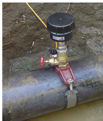
Figure 5. Permanent flow monitoring with WLM probe
