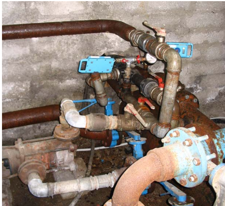
Figure 1.2 Uncontrolled extensions at the outlet of a booster.
